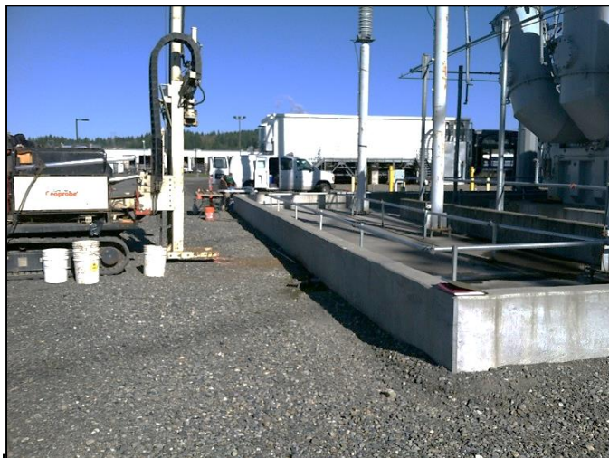
Figure 6 – Installing Well MW-1 by GSU#1 Containment Structure
