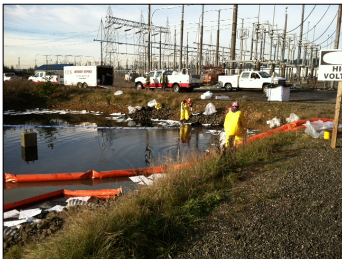
Figure 3 – Stormwater Pond Cleanup after GSU#3 Spill
