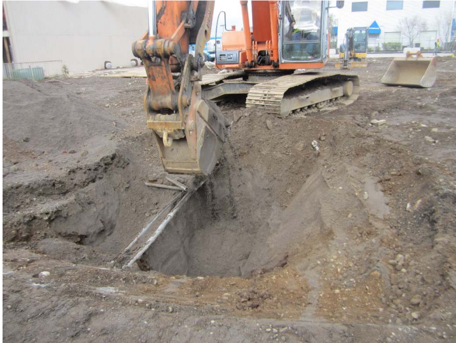
Photograph 7: Electrical conduit encountered during excavation of test pit TP5. Photograph taken facing west.
