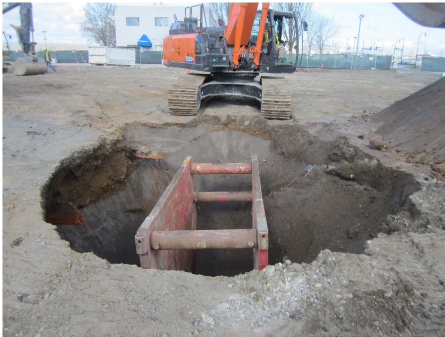
Photograph 4: Test pit TP2. A trench box was used to limit sidewall sloughing. Photograph taken facing west.
