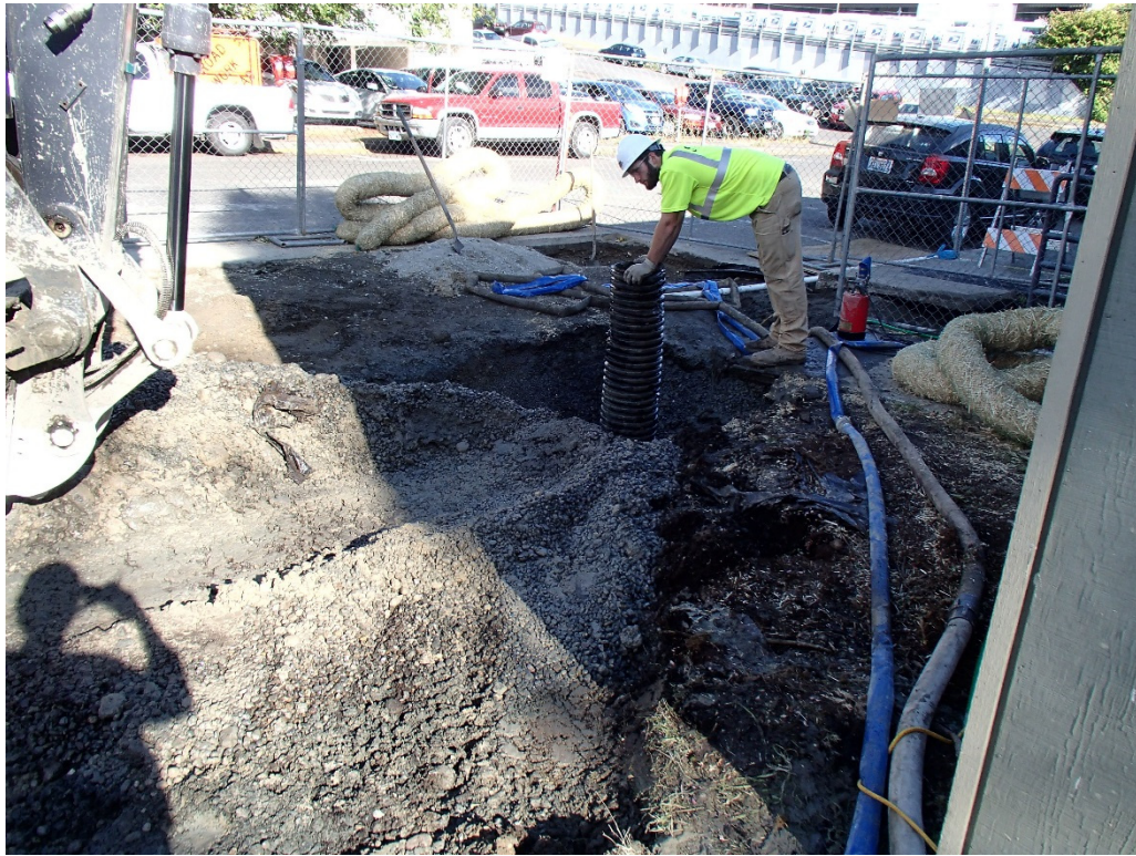
Photograph 19. Construction of Temporary Dewatering Sump North of Main Excavation Area and Dewatering Pumps
