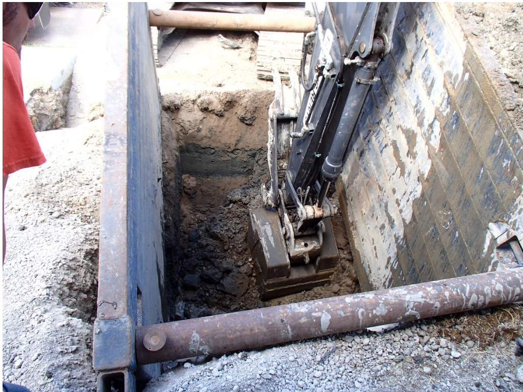
Photograph 16. Excavation Cell within Trench Box
