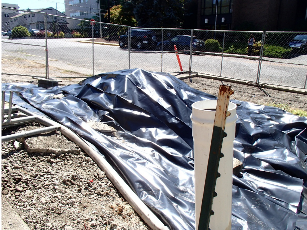
Photograph 9. Stockpiled Utility Trench Excavation Soil
