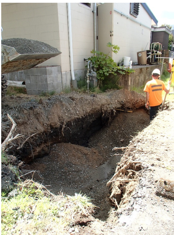
Photograph 4. Backfill Placement in Secondary Excavation Area
