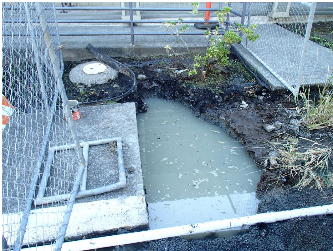
Photograph 10. Artesian Groundwater at North End of Utility Trench
