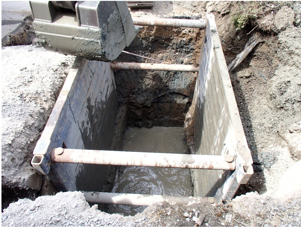
Photograph 17. Typical Final Depth of Main Excavation Cell and Groundwater Intrusion
