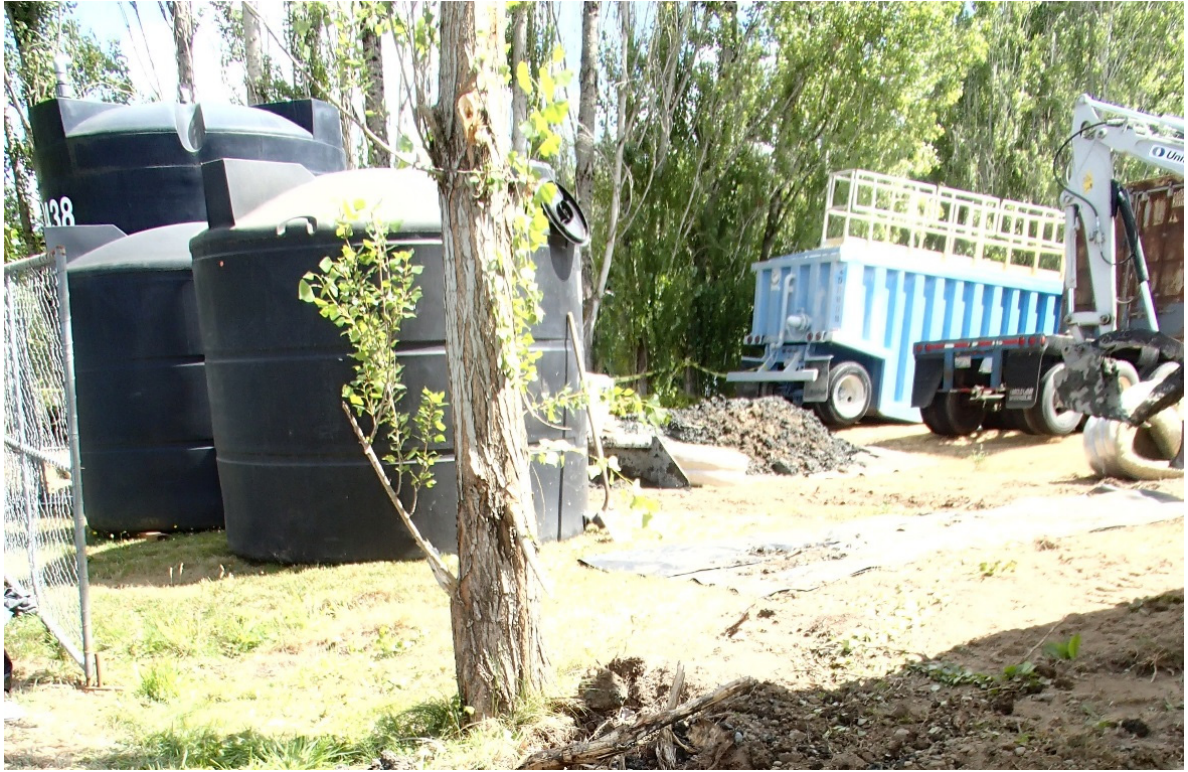
Photograph 29. View of 20,000-Gallon Settling Tank and Three Dewatering Water Treatment Tanks
