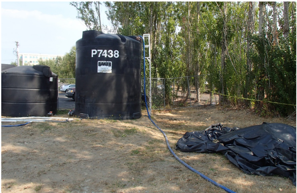
Photograph 30. Transfer of Dewatering Water from Settling Tank to Treatment Tank
