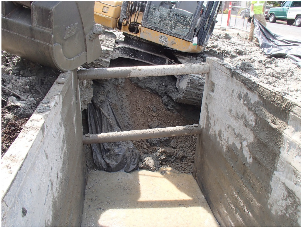
Photograph 25. Unstable Gravel Backfill in Previously Excavated Area
