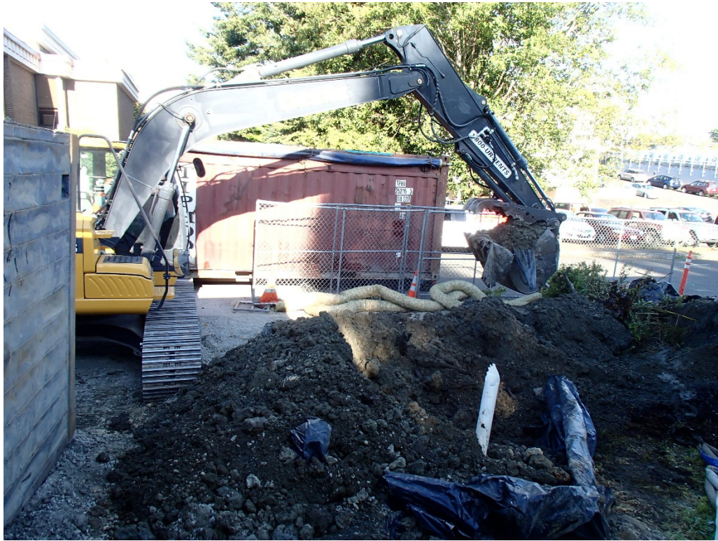
Photograph 15. Direct Loading Soil to Intermodal Bin
