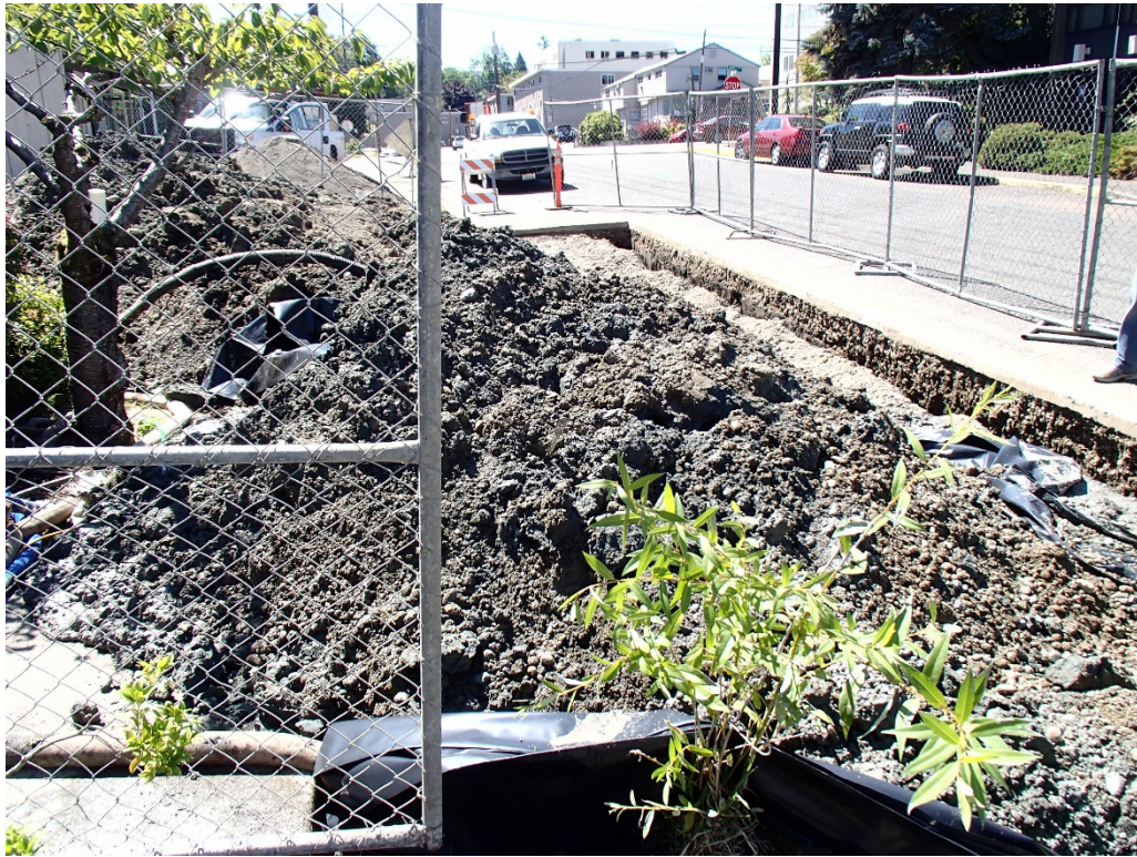
Photograph 11. Sand Backfill in Utility Trench
