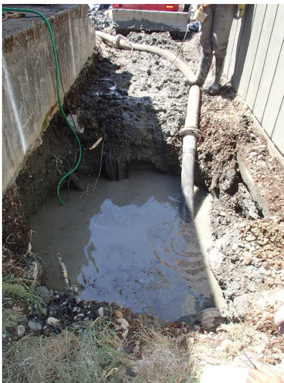
Photograph 22. Delivery of CDF Backfill via Pump Truck
