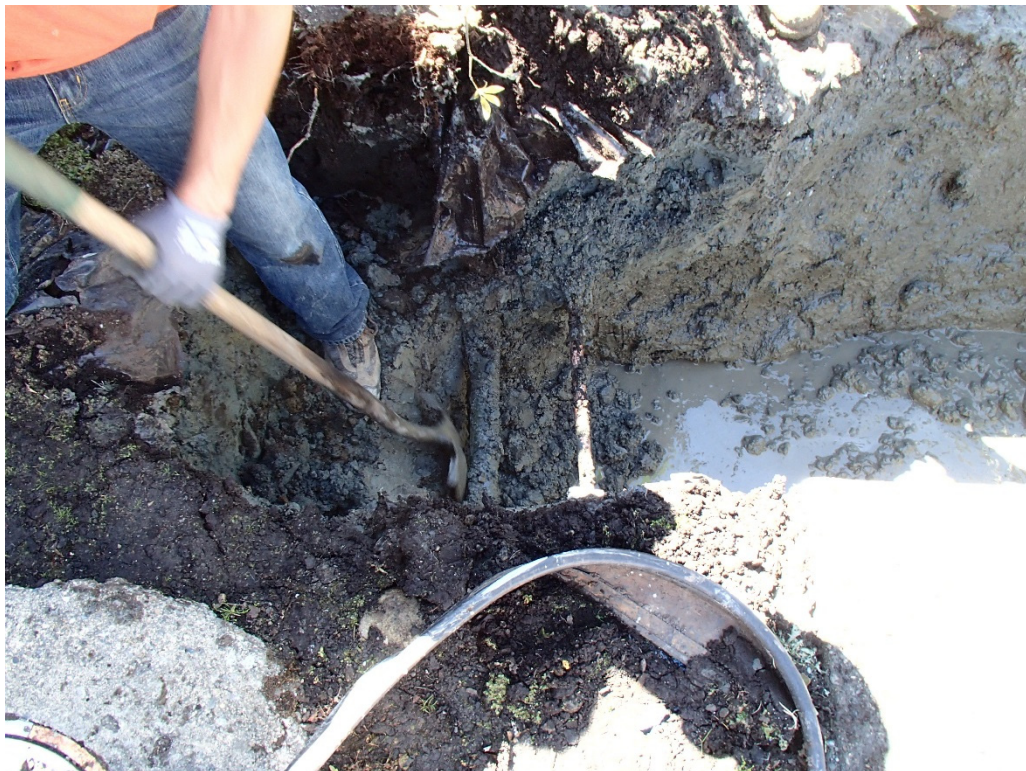
Photograph 8. Exposed Gas and Water Line North of Main Excavation Area and Groundwater Intrusion
