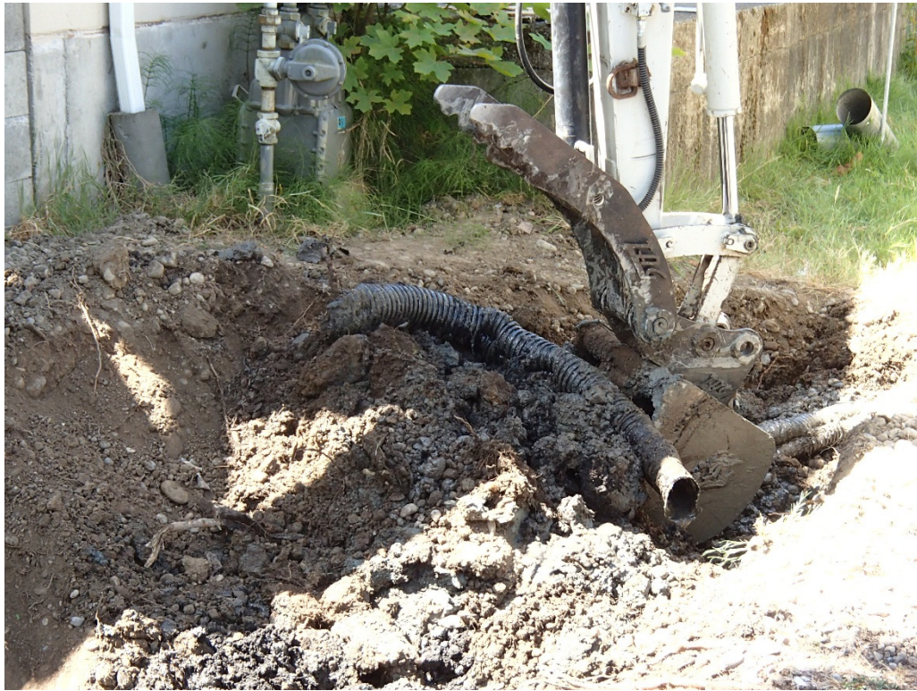
Photograph 1. Corrugated Drain Pipe in Secondary Excavation Area
