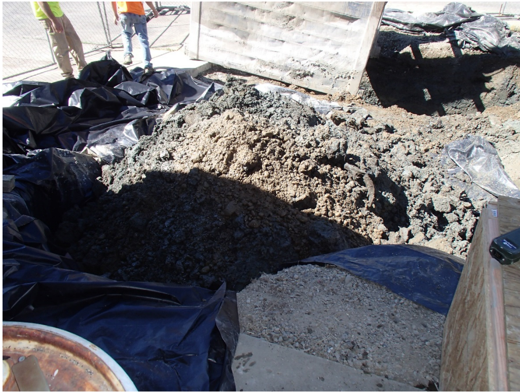
Photograph 23. Stockpiled Main Excavation Soil on Cured CDF Backfill
