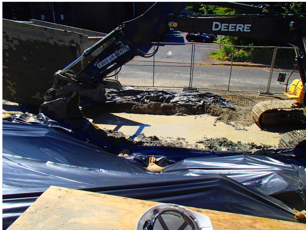
Photograph 24. Main Excavation Cell Backfilled with CDF and Stockpiled Main Excavation Soil
