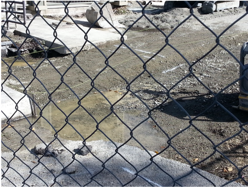
Photograph 31. Groundwater Seep After Final Main Excavation Backfill (Prior to Restoration)
