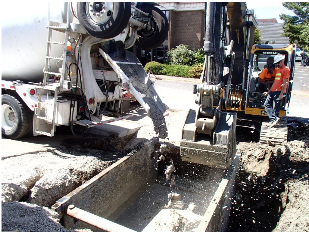
Photograph 18. Delivery of Controlled-Density Fill (CDF) Backfill via Truck Chute
