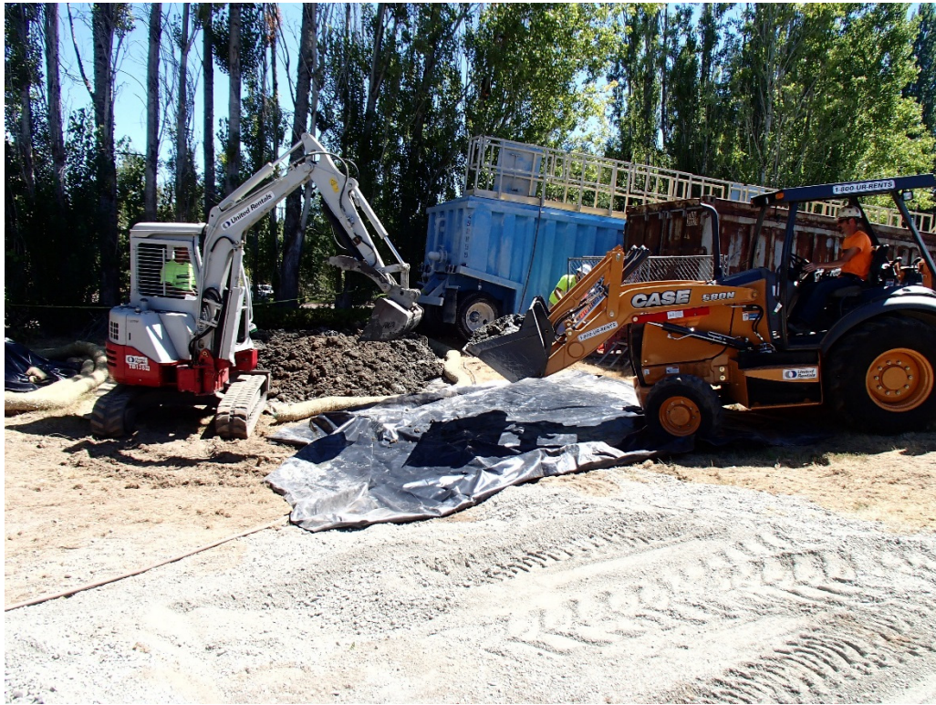
Photograph 13. Loading of Secondary Excavation Soil to Intermodal Bin
