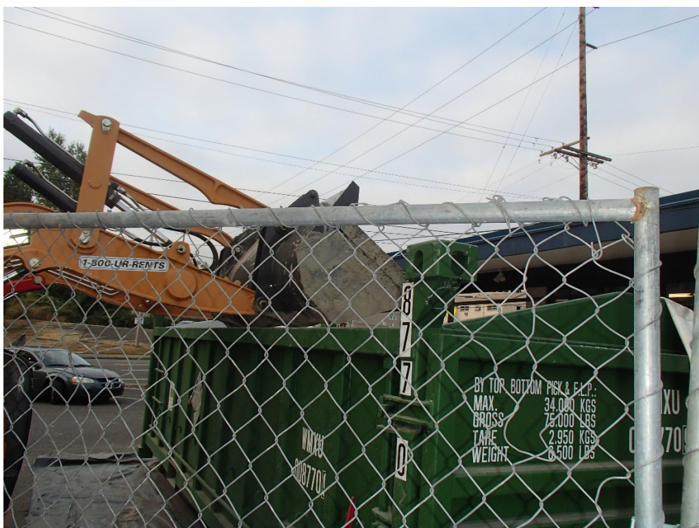
Photograph 28. Transfer of Soil to Hazardous Waste Bin
