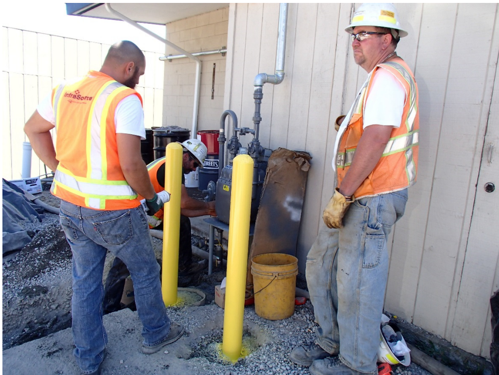
Photograph 12. Installation of New Gas Meter
