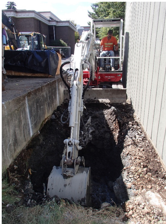
Photograph 20. Open Trench Alley Excavation
