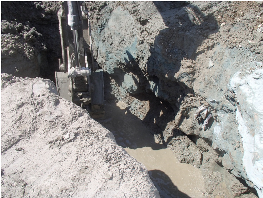
Photograph 27. Final Main Excavation Between Cured CDF Cells
