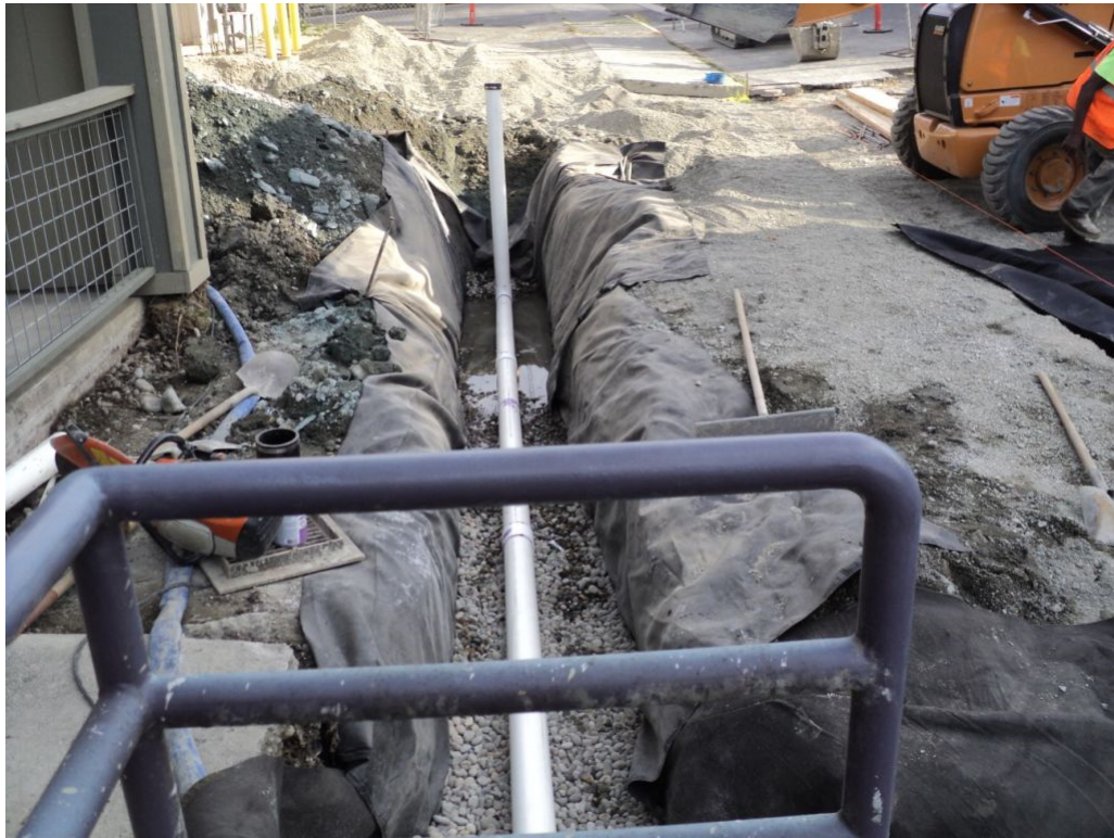
Photograph 33. French Drain and Conveyance Pipe to Sampling Access Standpipe
