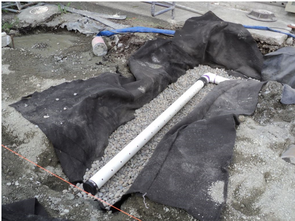
Photograph 32. Installation of Perforated Pipe French Drain North of Main Excavation Area
