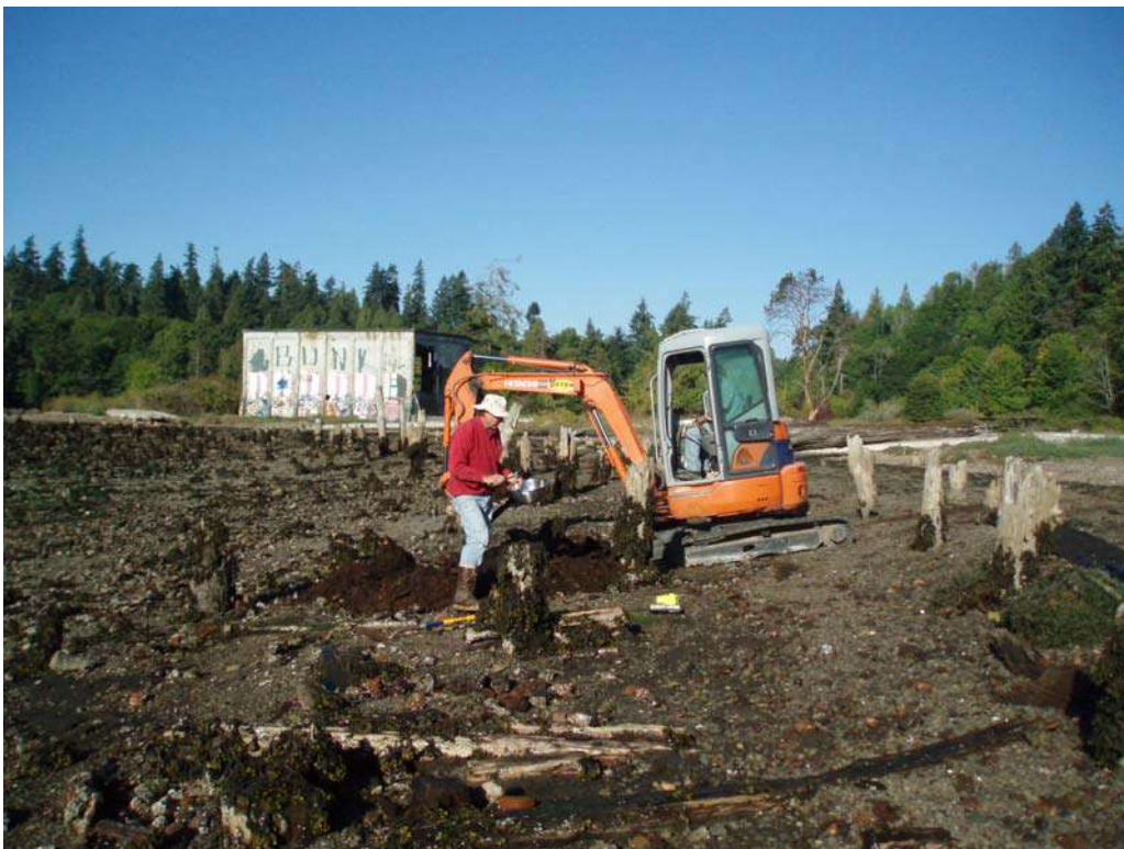
Photograph 8 – Test pit excavator at Test Pit 2
