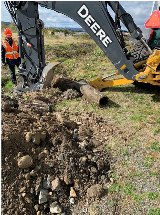
Photograph 3. Piece of pipe removed during excavation of TP-2.
