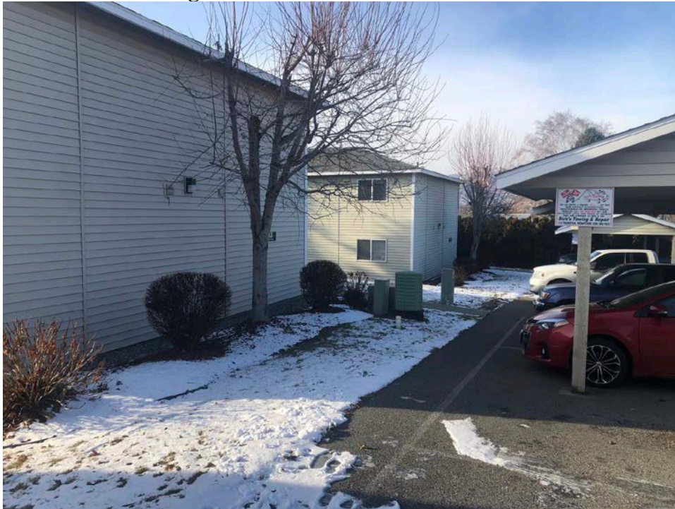
Photo 2: North side of buildings 581 and 583 - from the northeast.
