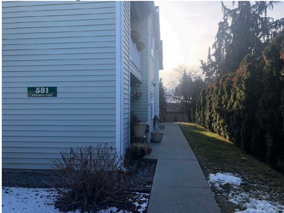
Photo 3: West side of building 581 - from the north.
