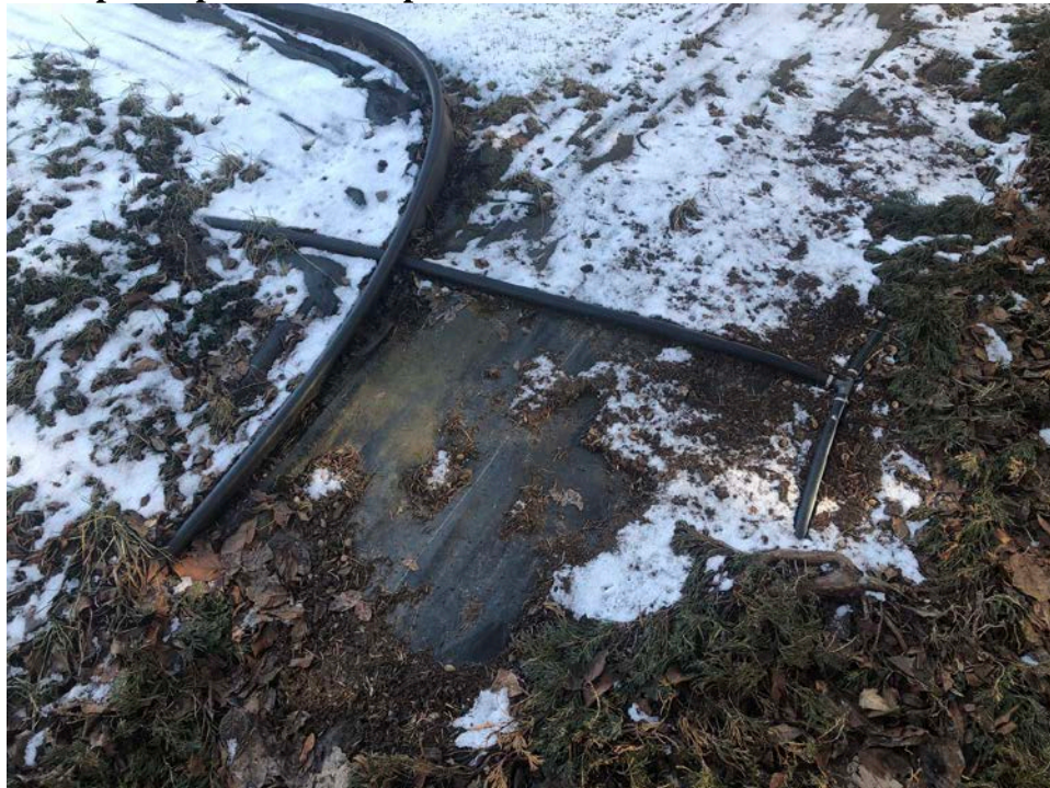
Photo 4: Close-up of exposed landscape fabric at southern end of area between 581 & 583.
