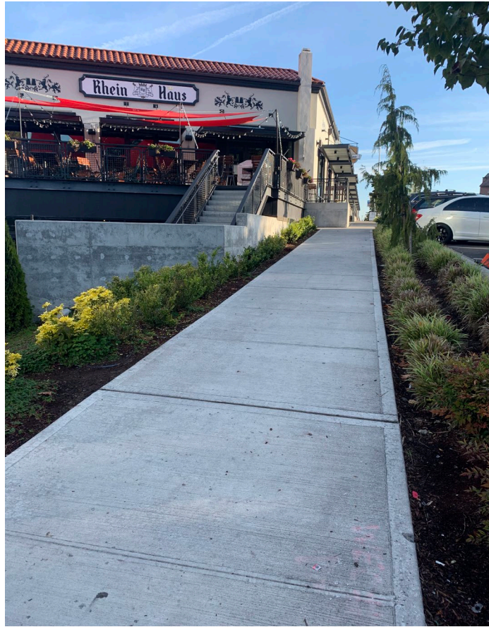
Photograph 9: View looking NE along Division Ave.
