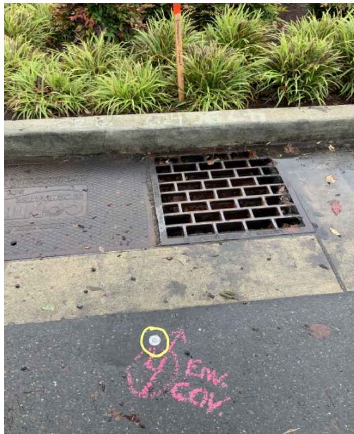
Photograph 6: Pavement Cap Monument "C" offset 4-feet from capped rebar at stake.
