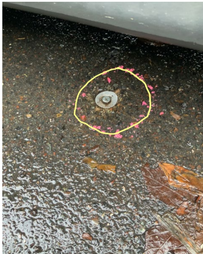
Photograph 4: Pavement Cap Monument "B".
