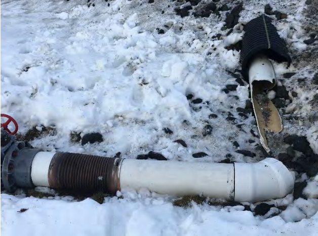
Before Header Replacement near N-33
