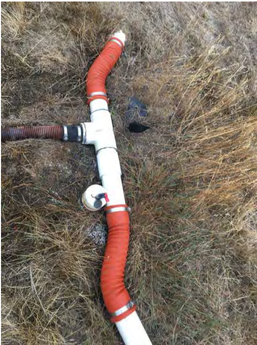
After 3" hose replacement at E-39
