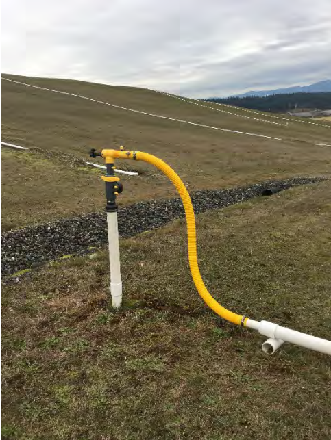
N-44 after QED wellhead replacement
