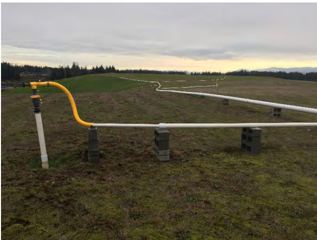
E-42 after QED wellhead replacement
