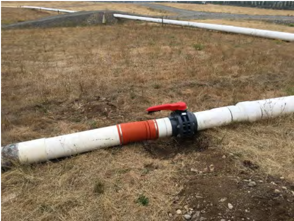
Before E-37 Header Installation
