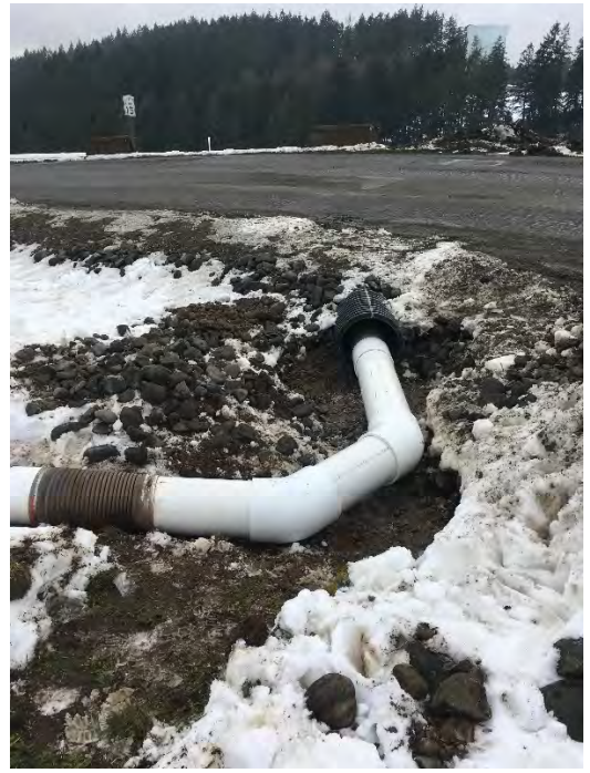
After Header Replacement near N-33
