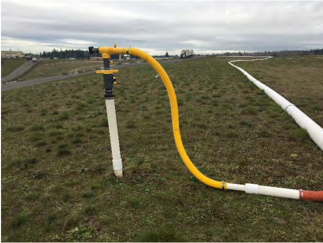
N-36 after QED wellhead replacement
