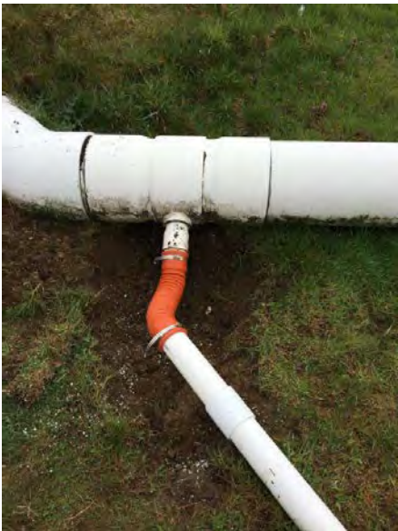
After hose replacement at N-5
