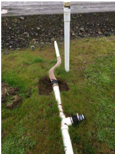
Before hose replacement at N-60
