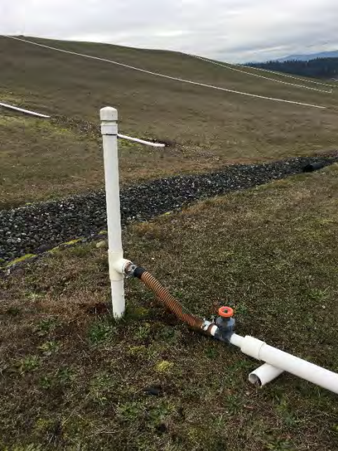
N-44 prior to QED wellhead replacement
