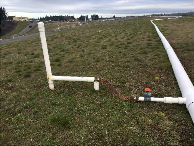
N-36 prior to QED wellhead Replacement
