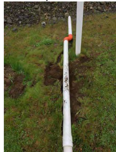
After hose replacement at N-60
