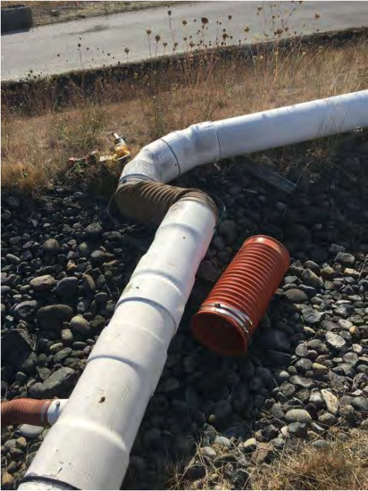
Before 10-in. hose replacement at E-26
