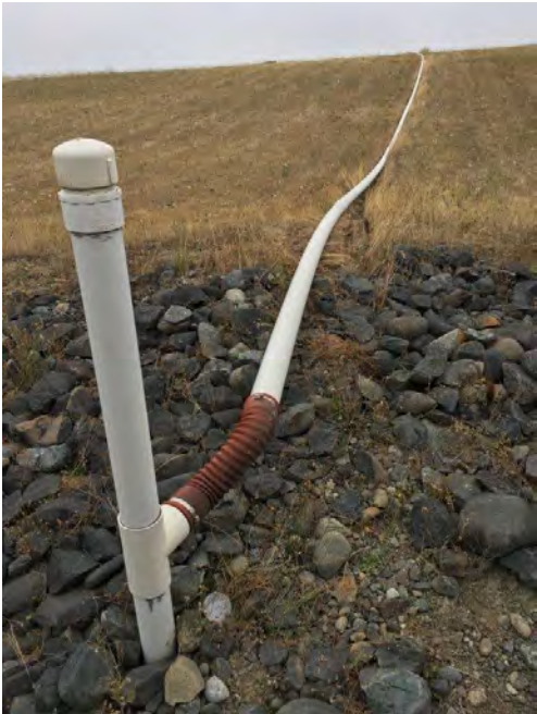
After N-56 repairs facing N
