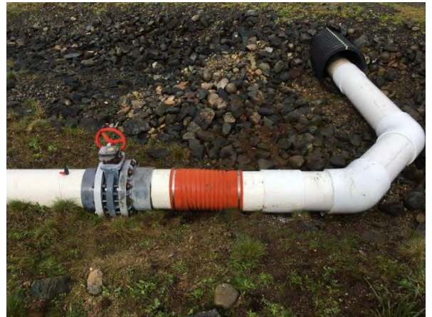
After hose replacement at N-33
