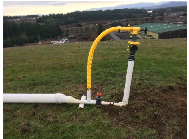
E-28 after QED wellhead replacement
