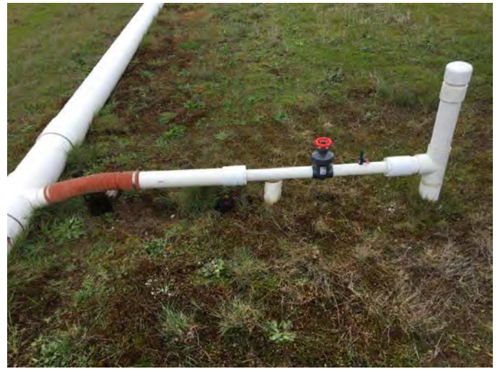
After hose and valve replacement at N-20
