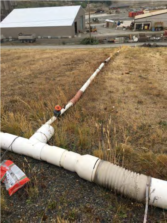
Before N-56 repairs facing S
