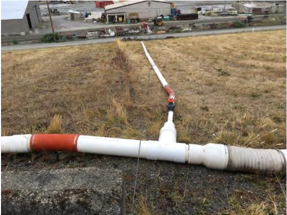
After N-56 repairs facing S
