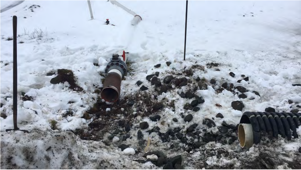
Before Header Replacement near N-33
