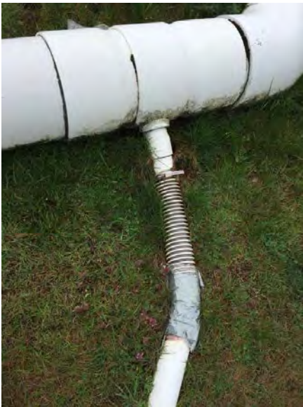
Before hose replacement at N-5
