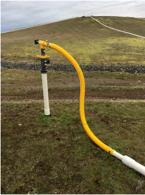
N-37 after QED wellhead replacement
