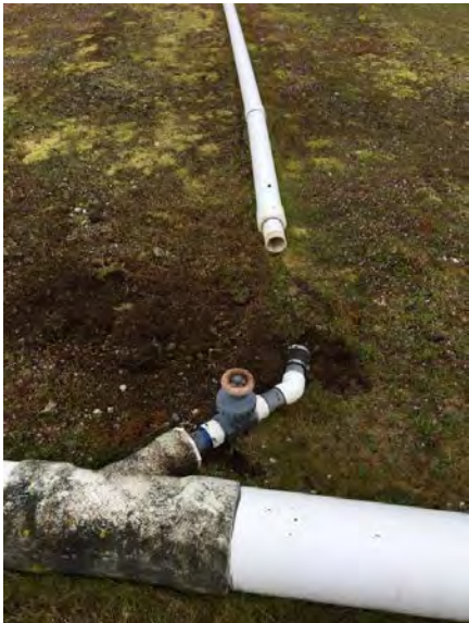
Before hose replacement at E2B
