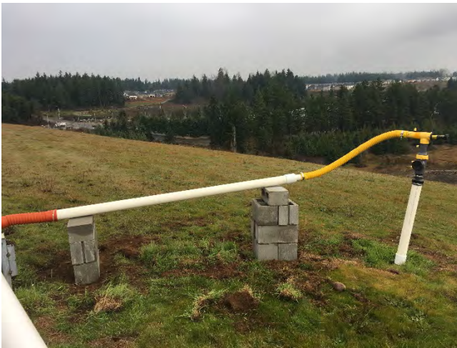
E-29 after QED wellhead replacement
