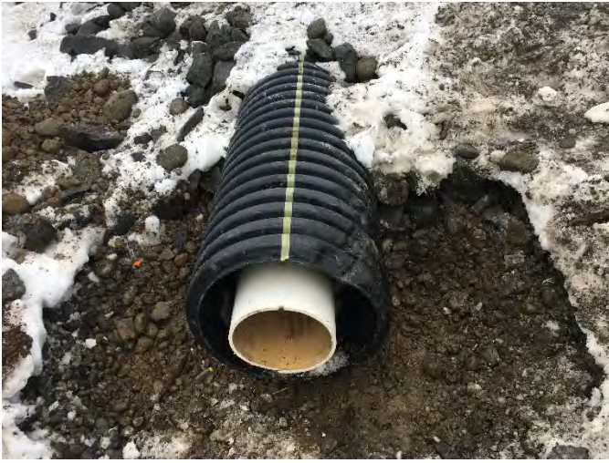
Before Header Replacement near N-33
