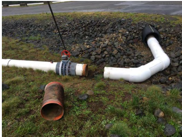
Before hose replacement at N-33
