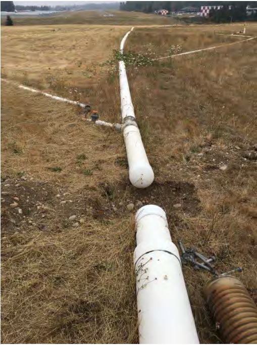
Before E-37 Header Installation
