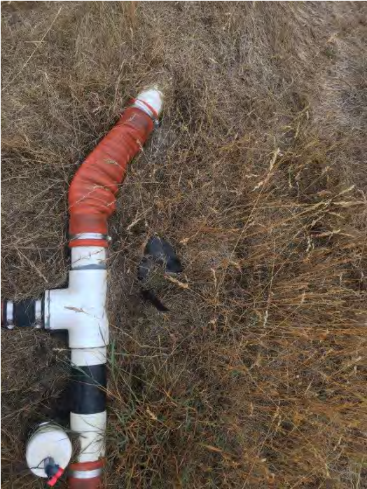
Before 3" hose replacement at E-39
