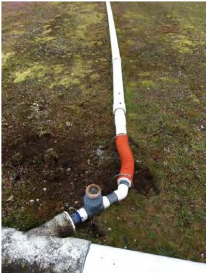
After hose replacement at E2B
