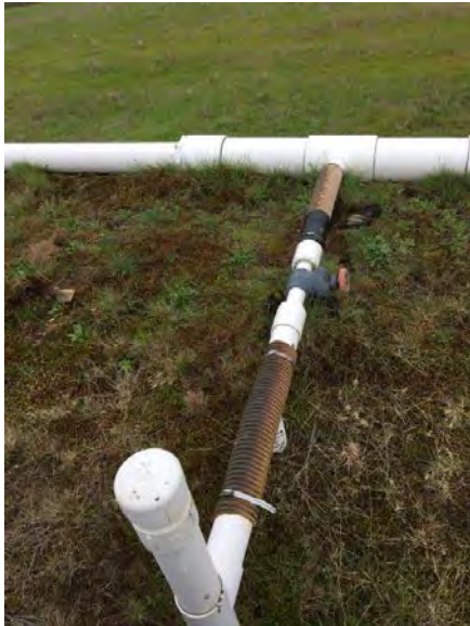
Before hose and valve replacement at N-20
