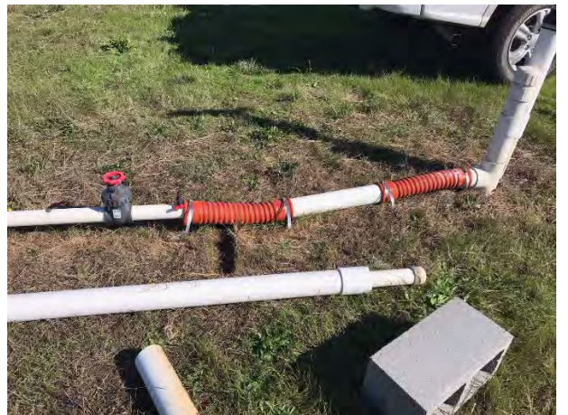
Hose replacement at E-43
