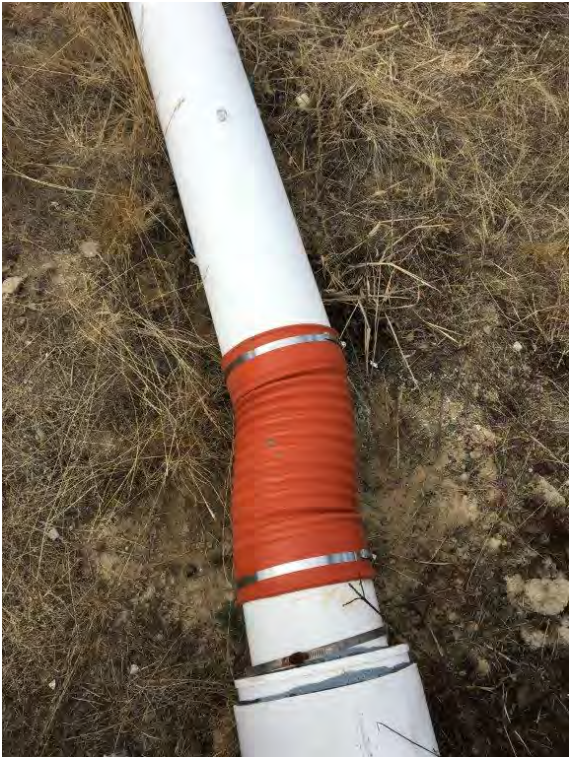
After 8-inch hose replacement at N-4
