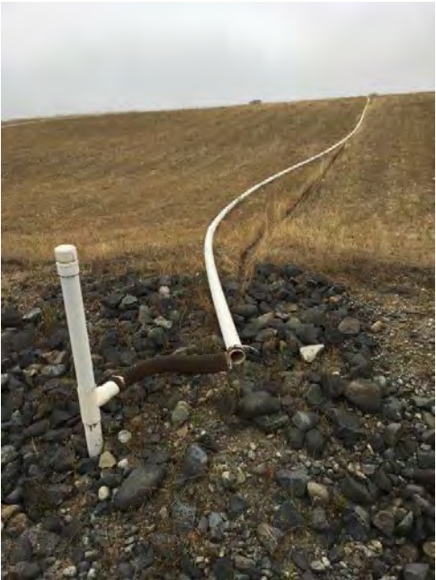
Before N-56 repairs facing N
