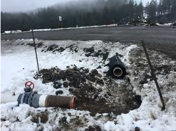
Before Header Replacement near N-33
