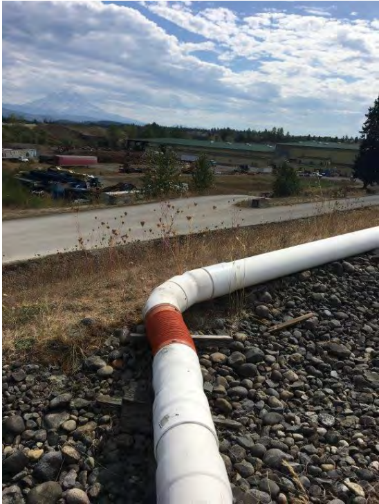
After 10-in. Hose replacement at E-26
