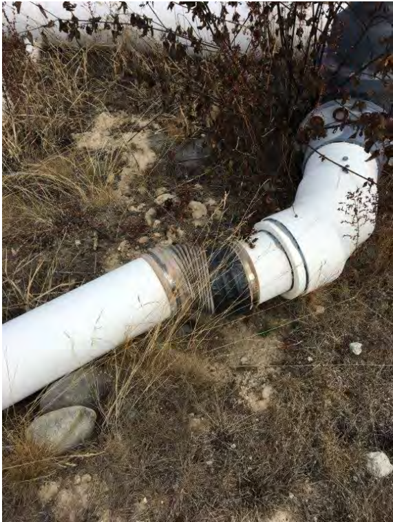
Before 8-inch hose replacement at N-4
