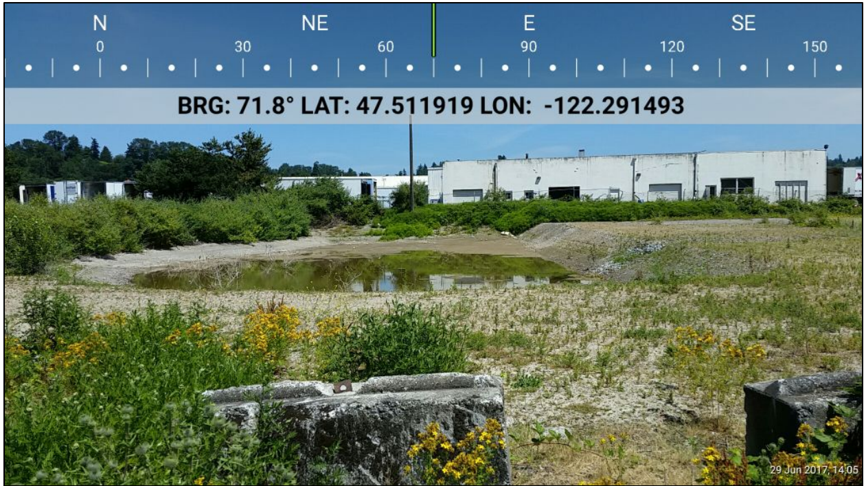
Figure 8. Conditions in central part of project; view is to the east.
