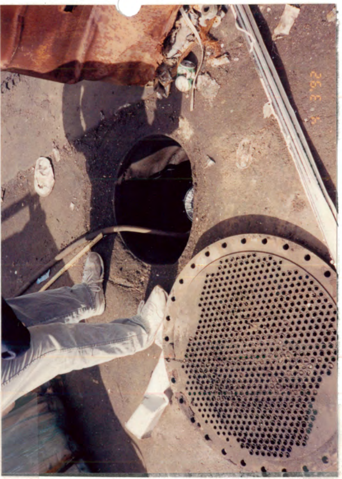
Close up of drain just east of Boiler Building. (Same location 376 & 37)
