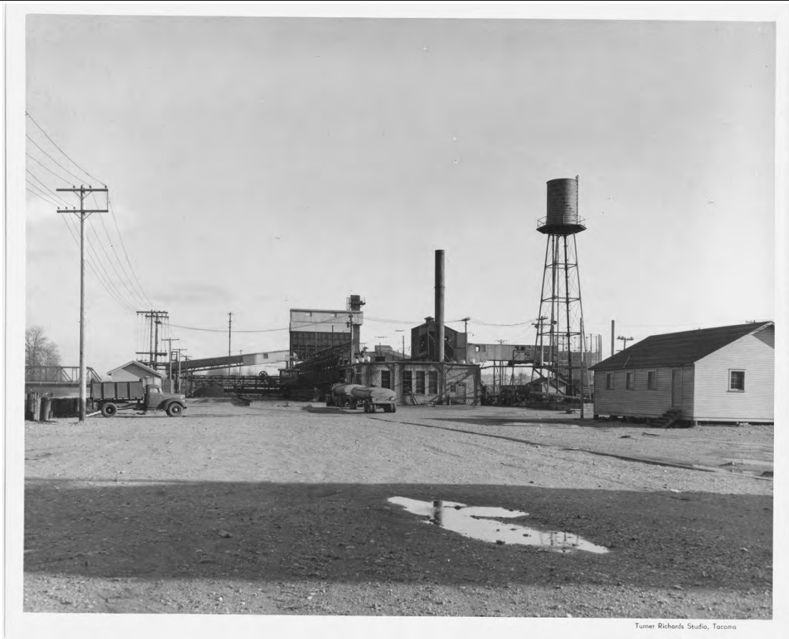
Photograph 5. “Coke plant interior and exterior for Wilkeson Products. On May 28, 1943, the first coke oven was charged at this site. After its success six more ovens were charged the following day. During the first week of June 1943, operations began at this million-dollar Pacific Northwest coke plant.” (Richards Studio D17139-1; image date: 1944-03-09)
