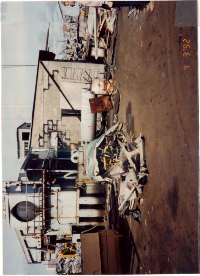
View of Boiler Building looking west Drum is located next to the Rusty Drum in front
