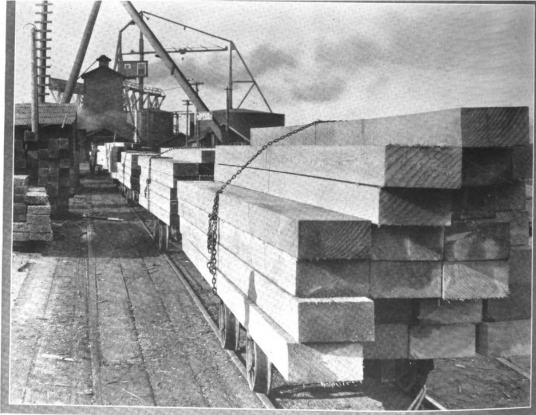
Bridge stringers as they arrive at the creosoting plant for treatment. The daily capacity of this plant is 40,000 feet is the both will. Photograph 1. "Bridge stringers as they arrive at the creosoting plant for treatment. The daily capacity is 40,000 feet." (American Lumberman, 1921)
