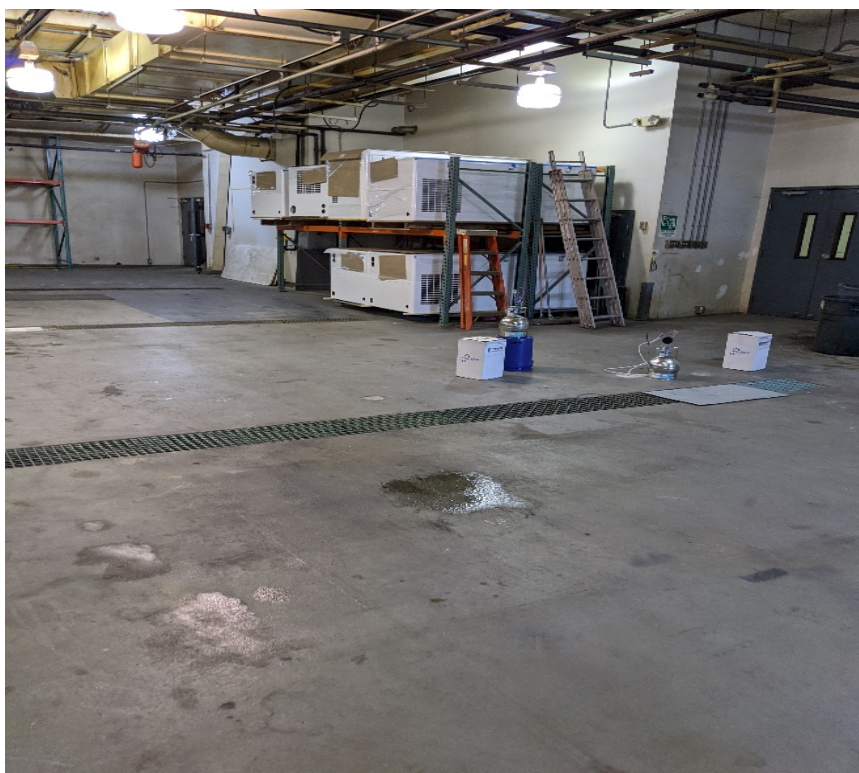
Photograph 6: Date: March 11, 2020 time: 12:52. Sample location and setup of SV-3 and IA-3 and patched flooring in background in the eastern section of the UMC building.
