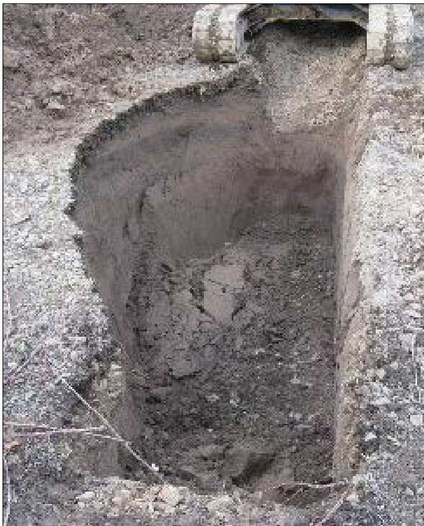
Figure 3. Photo of Trench CW-10 wall collapse (Photo by PGS).
