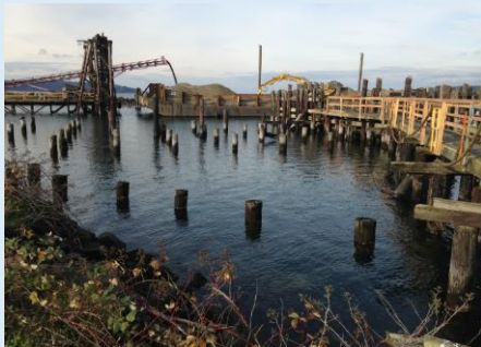
In-water structures before cleanup.
