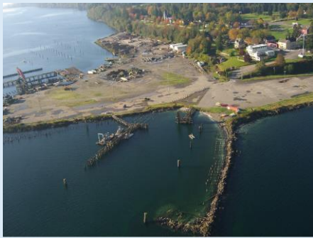
Upland Mill site during in-water cleanup.
