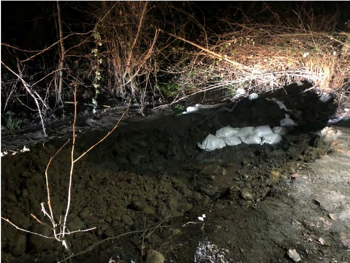
Photograph 5. Midexcavation, evening of 3/6/20. Sandbags set against soil berm below culvert to maintain separation from stormwater drainage (looking southeast).
