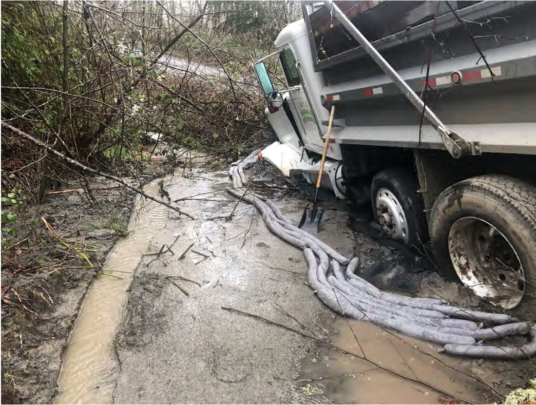
Photograph 2. View of stormwater bypass (left side) and absorbent socks containing diesel spill on 3/6/2020 (looking south).
