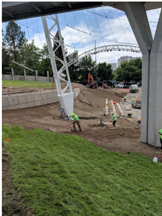
Photograph 6. Installing soil cover and sod.
