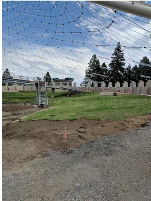
Photograph 5. Sod installed over the 12-inch cover soil.
