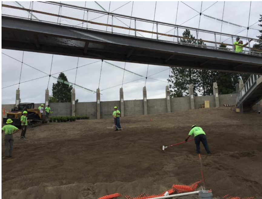
Photograph 3. Raking out the cover soil.
