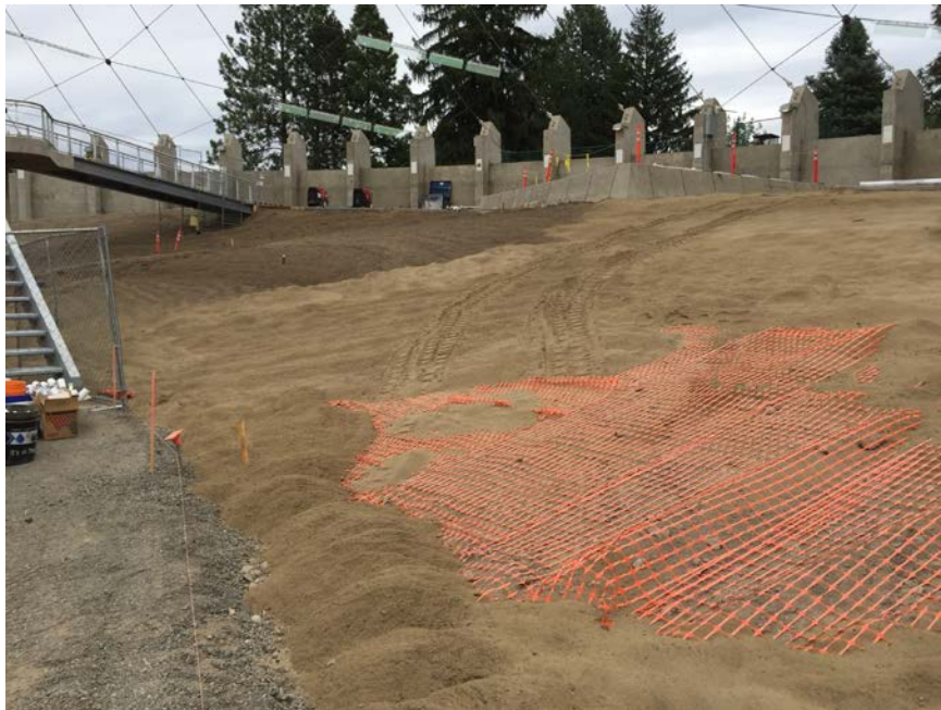
Photograph 4. Cover soil was deployed in two 6-inch lifts. The darker upper 6 inches was a turf builder product that had increased organics to enhance vegetation growth.
