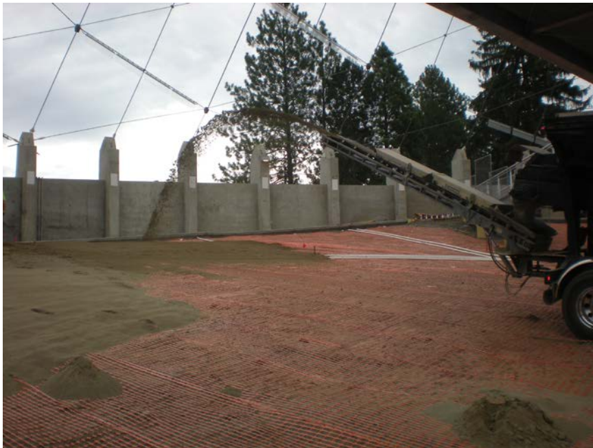
Photograph 2. Placement of cover soil over the orange construction fencing.
