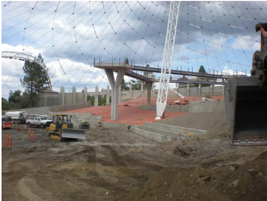
Photograph 1. Installation of the orange construction fencing , used as a visual indicator.
