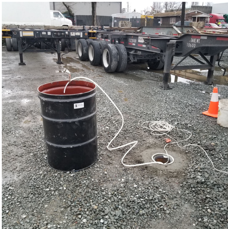
Photograph 2: View developing monitoring well SM-MW2.
