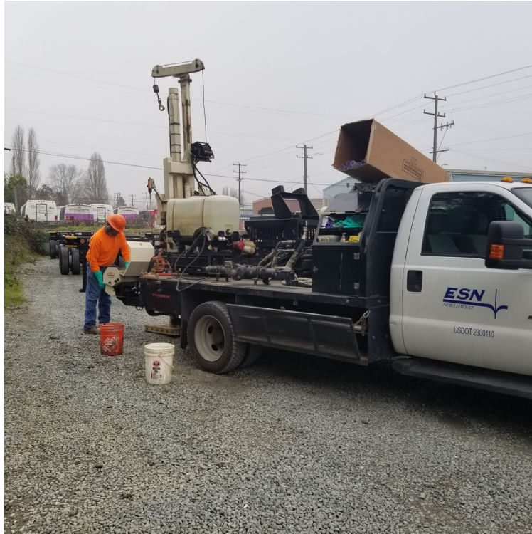
Photograph 1: View of drill rig set up on a monitoring well location.
