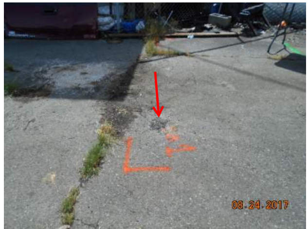
Photograph 8. View of typical soil boring plugging capped with asphalt patch.
