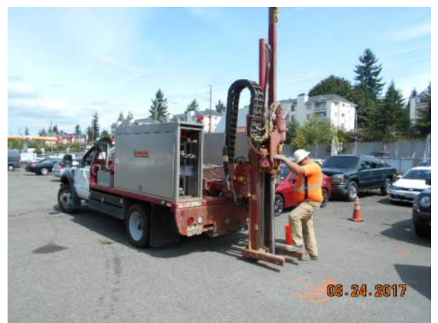
Photograph 6. Installation activities for temporary vapor monitoring point TVMP-2, in the footprint of the proposed building.
