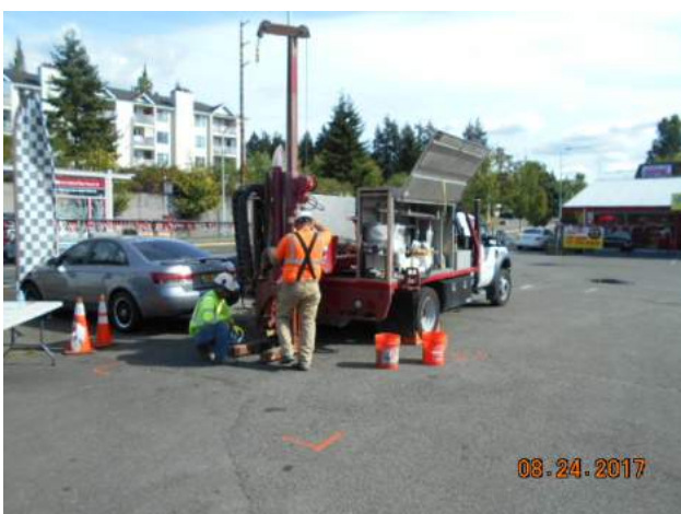
Photograph 5. Installation location for SB-5, within the former underground PST tankpit.
