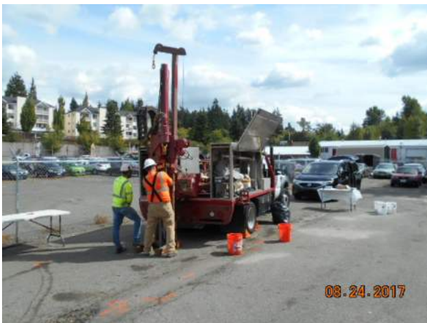
Photograph 3. Installation activities for soil boring SB-3, in the vicinity of the former greenhouse.
