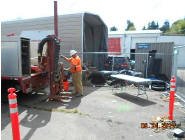
Photograph 1. View of installation activities associated with soil boring SB-1.
