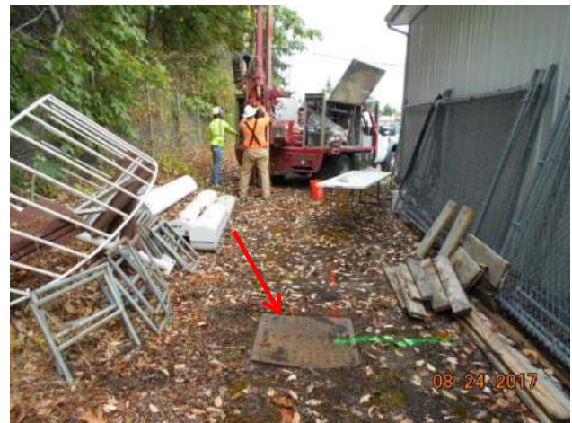
Photograph 4. Installation activities for soil boring SB-4, adjacent to the auto repair bays. Note the sump and underground line locations.
