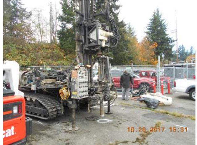
Photograph 2. Installation activities associated with soil boring SB-6, within proposed building footprint.
