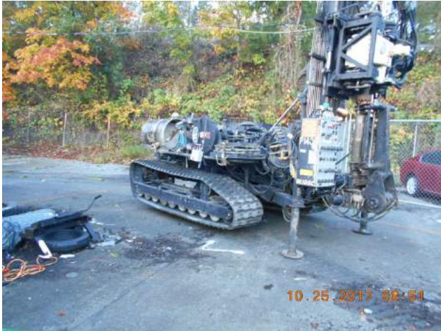
Photograph 1. View of installation activities associated with soil boring TSB-1.
