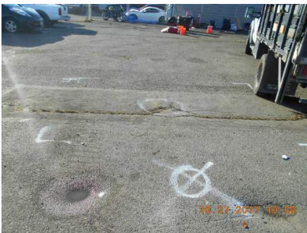
Photograph 5. View of typical soil boring plugging capped with concrete patch.
