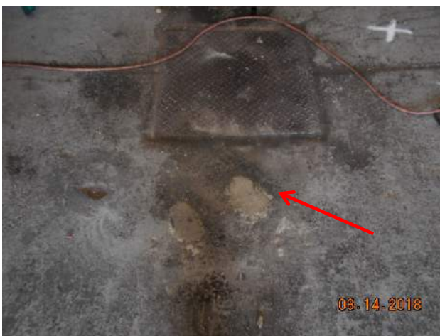
Photograph 5. View of typical plugged soil boring.
