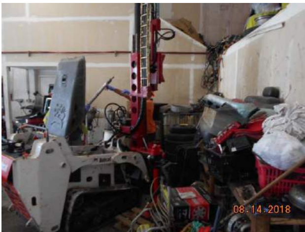
Photograph 3. Installation activities for soil boring B-6, adjacent to the waste storage area in the rear of Bay 3.
