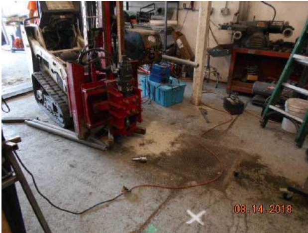
Photograph 1. View of installation activities associated with soil boring B-3.
