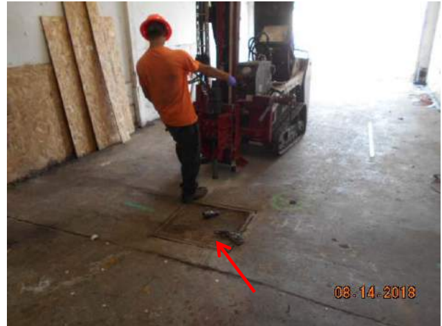
Photograph 4. Installation activities for soil boring B-8, adjacent to the sump in Service Bay 5.
