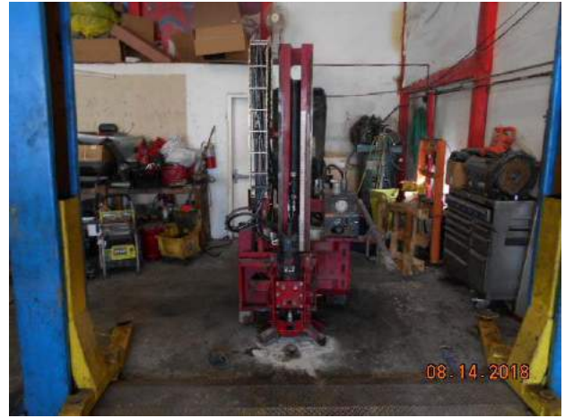
Photograph 2. Installation activities associated with soil boring B-4.
