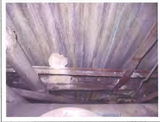
Photo 22. Asbestos containing debris from above damaged piping resting on siding.
