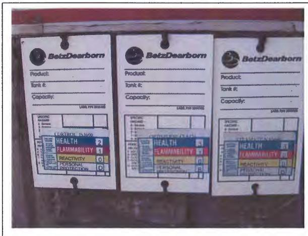
Photo 11. Chemical storage tank labels detailing contents.
