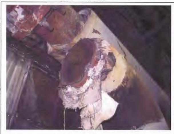
Photo 20. Damaged asbestos containing piping.
