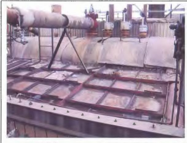
Photo 25. Asbestos containing piping in poor condition on the roof of Boiler 4. Water tank insulation under piping was non-detect for asbestos.
