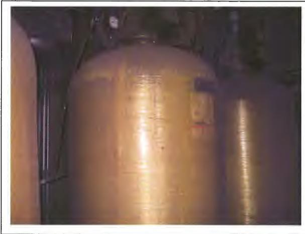
Photo 13. Water purification tanks located inside the Water Softening Room adjacent to the Hog Fuel Boiler House.
