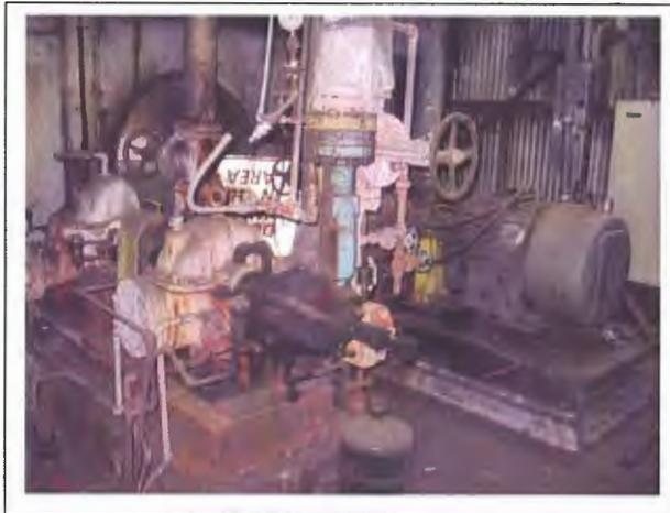
Photo 18. Generator system in the Hog Fuel Boiler House attached to asbestos containing high pressure steam piping system.
