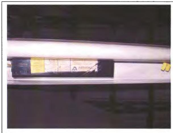
Photo 12. PCB containing fluorescent light ballast.
