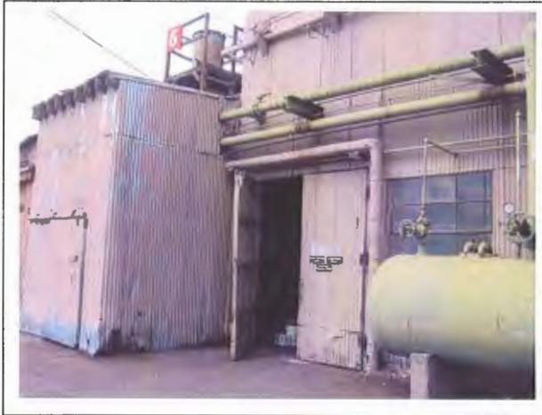
Photo 17. Asbestos containing piping (painted tan) adjacent to the green above ground storage tank can be seen penetrating the ground on the right.
