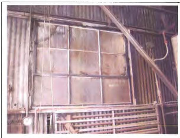
Photo 16. Asbestos containing window glazing, typical of the Hog Fuel Boiler House.
