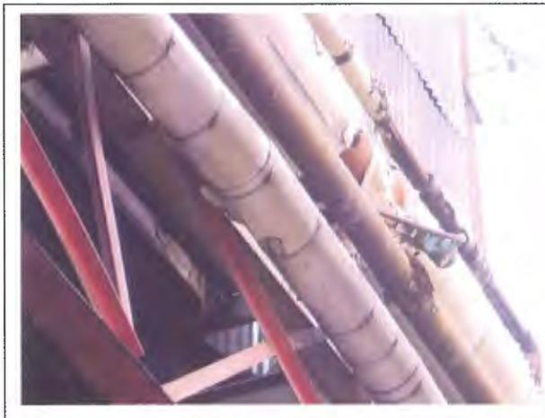
Photo 23. Asbestos containing piping on the exterior of the building. Damage to top two pipes has resulted in pieces falling off to the ground below as seen in Photo 24.
