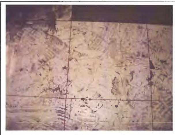
Photo 15. Asbestos containing vinyl tile in the bathroom of the Hog Fuel Boiler House.
