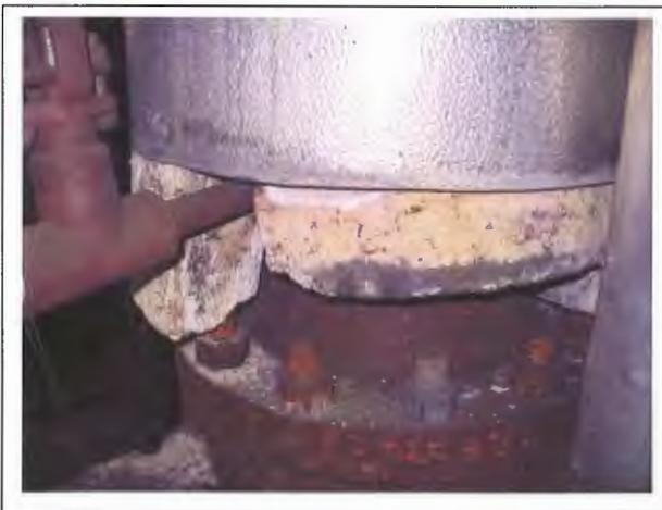
Photo 19. Asbestos containing pipe insulation and associated dust and debris underneath.
