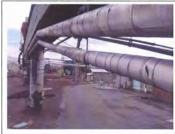
Photo 26. Piping running from the Hog Fuel Boiler House to other locations on the site.
