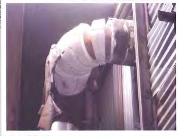
Photo 21. Asbestos containing piping in poor condition penetrating the siding of the Boiler Room of the Hog Fuel Boiler House.
