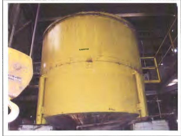
Photo 6. Caustic vat located inside the Caustic Storage Room of the Hog Fuel Boiler House. The contents of the caustic material are unclear.
