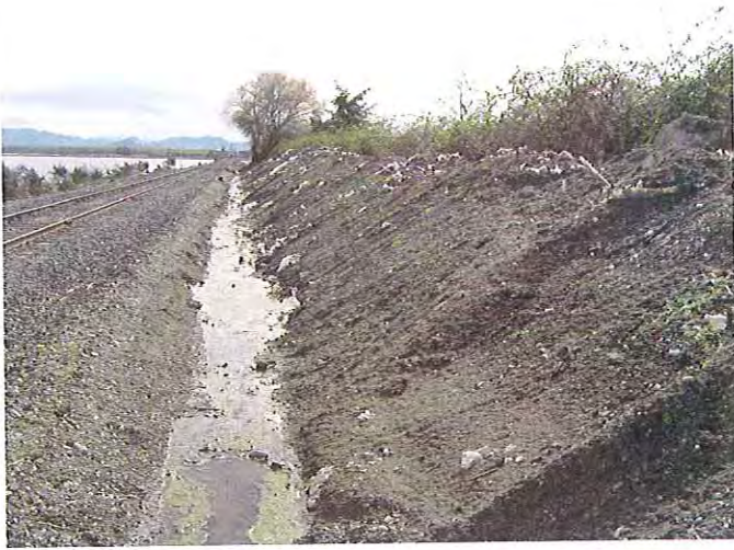
Photo 1: Drainage ditch on northeast side of landfill looking southeast
