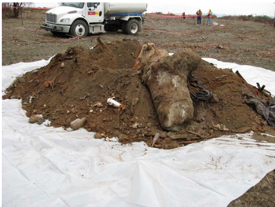
Photograph 6 Tank at TP-G-2.
