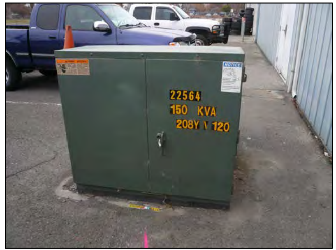
Photograph 2: A pad-mounted transformer near the northeast corner of the vehicle maintenance shop.
