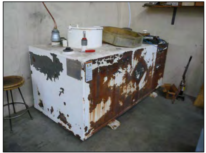
Photograph 20: the 250-gallon waste oil AST at the interior southwest corner of the shop.
