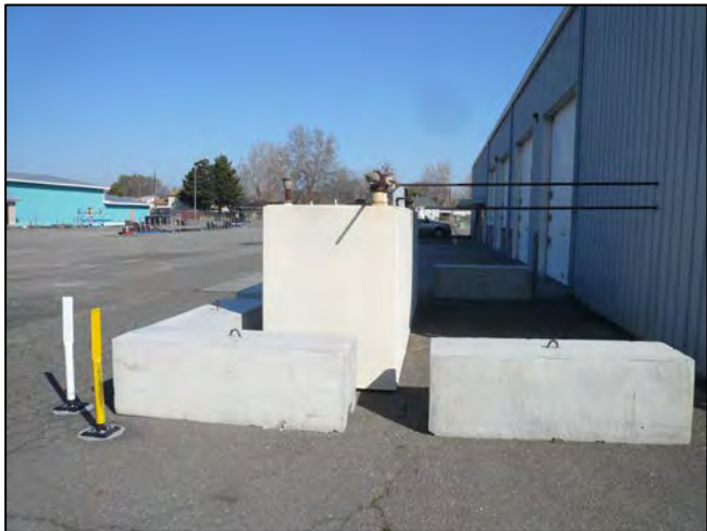
Photograph 21: View of the recently installed 2,930-gallon waste oil AST at the exterior southwest corner of the vehicle maintenance building.
