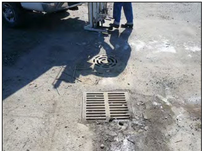
Photograph 5: View of the wash rack area.
