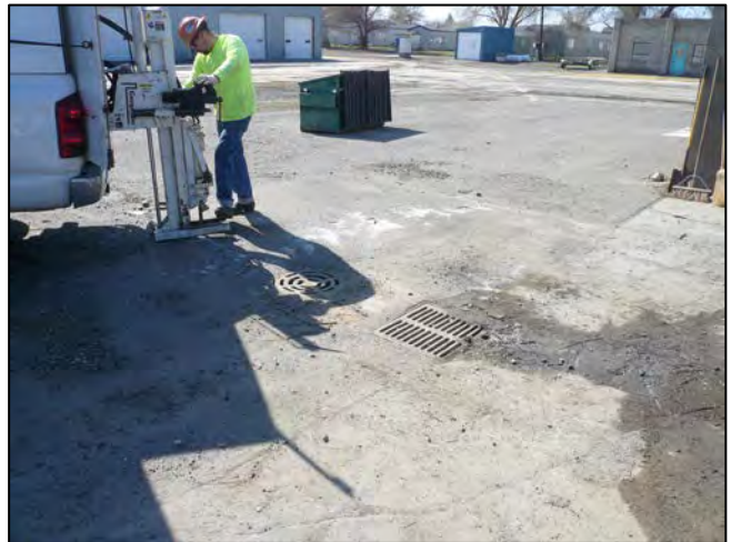
Photograph 4: Drilling near the wash rack east of the oil/lube building.
