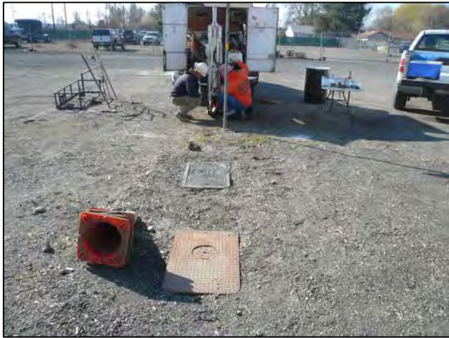
Photograph 1: View of the area surrounding the Waste Oil USTs.
