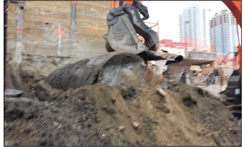
6. UST2 was removed form the subject property – Looking West
