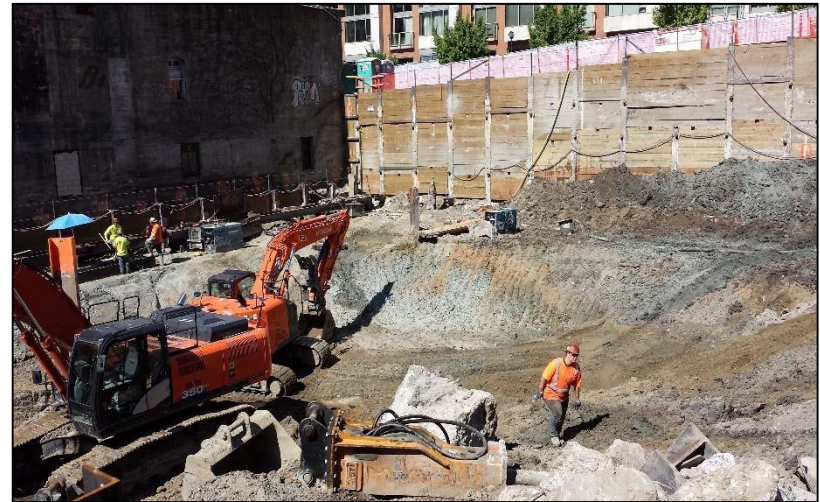
12. Clean native soil at the former elevator shaft and hydraulic hoist location in central portion of the subject property – Looking Northeast
