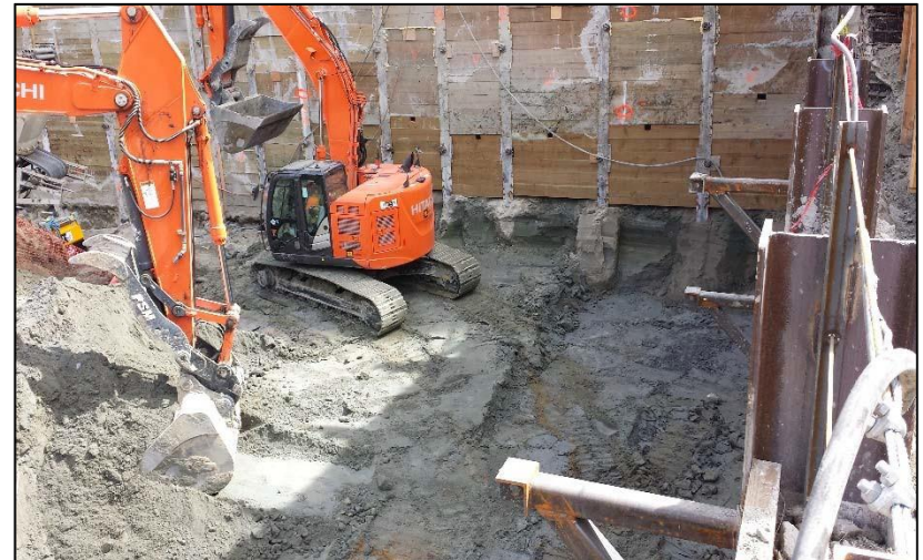
8. Clean native soil following excavation of contaminated soil at the former UST2 location In southwest portion of the subject property – Looking South
