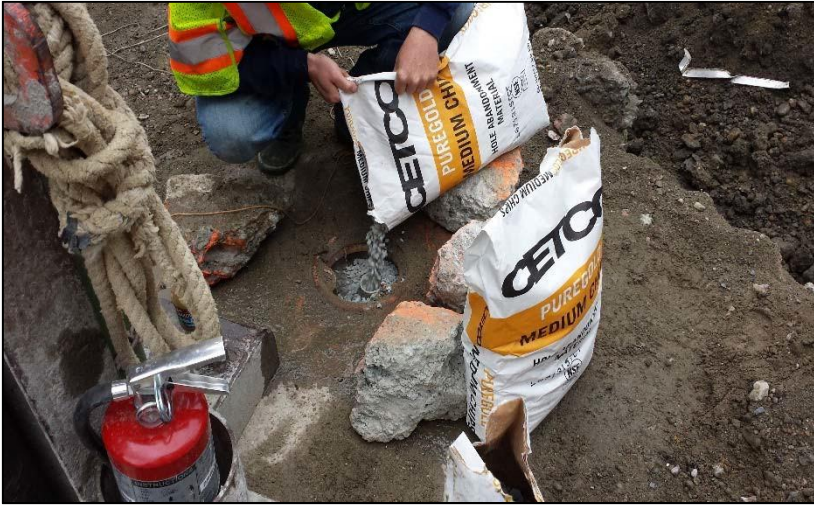
9. Monitoring wells decommissioning activities at the subject property
