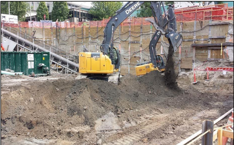
3. Contaminated fill soil excavation during construction - Looking Southeast
