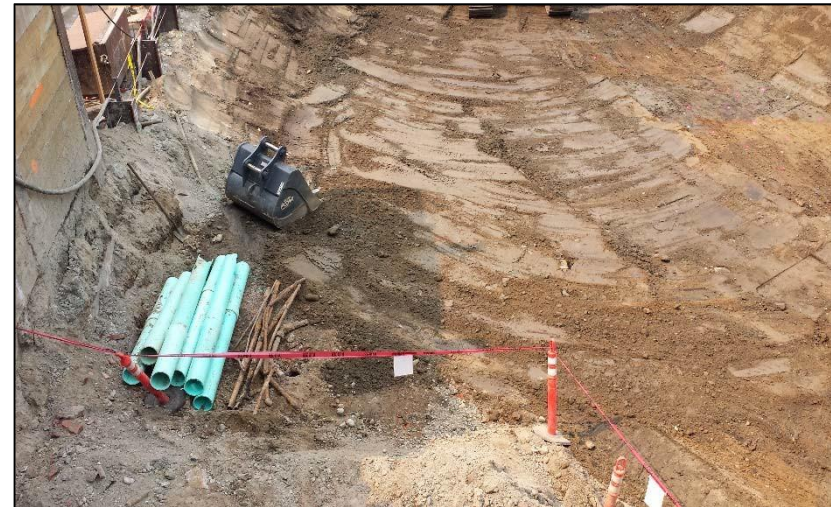
4. Non-contaminated soil underlying the contaminated fill soil excavated from the subject property - Looking North
