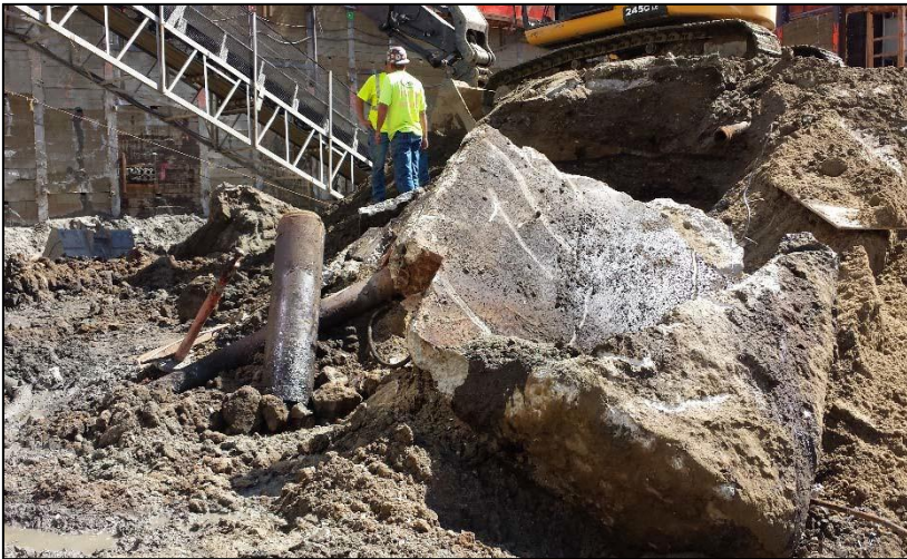
11. Excavation of former elevator shaft and hydraulic hoist – Looking South
