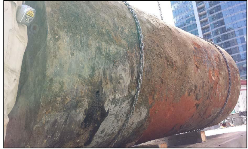
14. A small hole is visible in UST3 that was removed from the subject property
