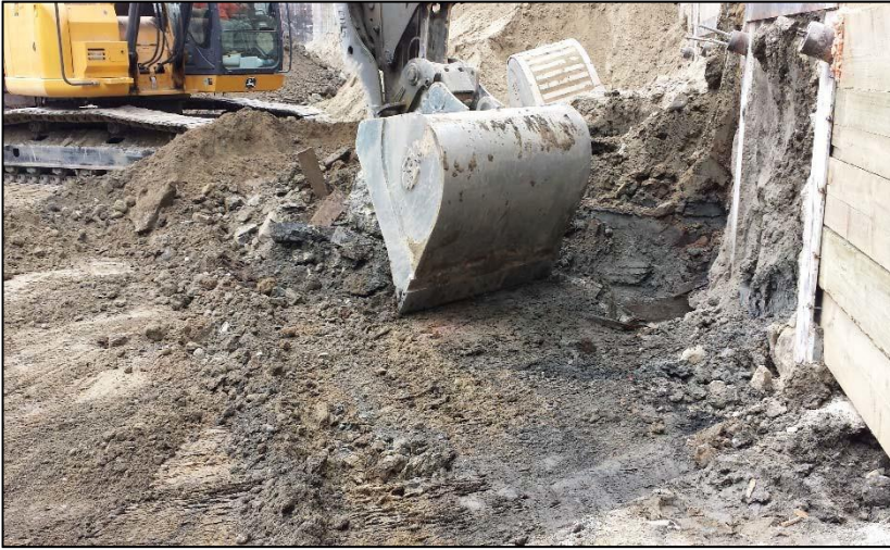
1. Contaminated fill soil in east portion of mass excavation - Looking North
