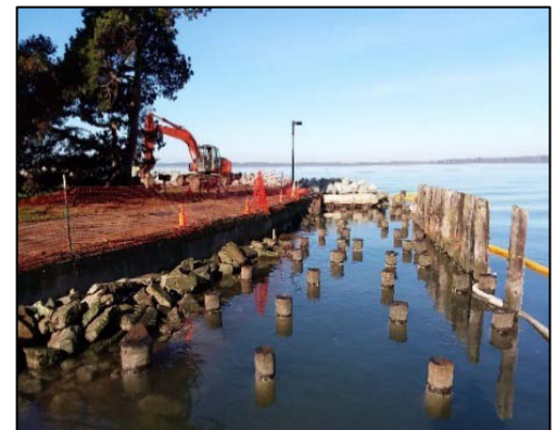
Public pier removal, October 2017
