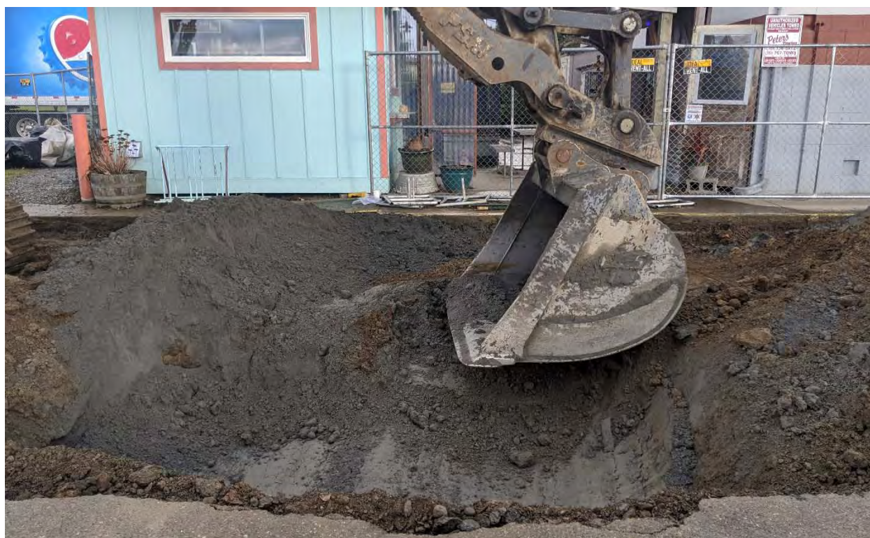
Figure 7. Photo of the former pump island excavation. Grey discolored soil had strong petroleum odors.
