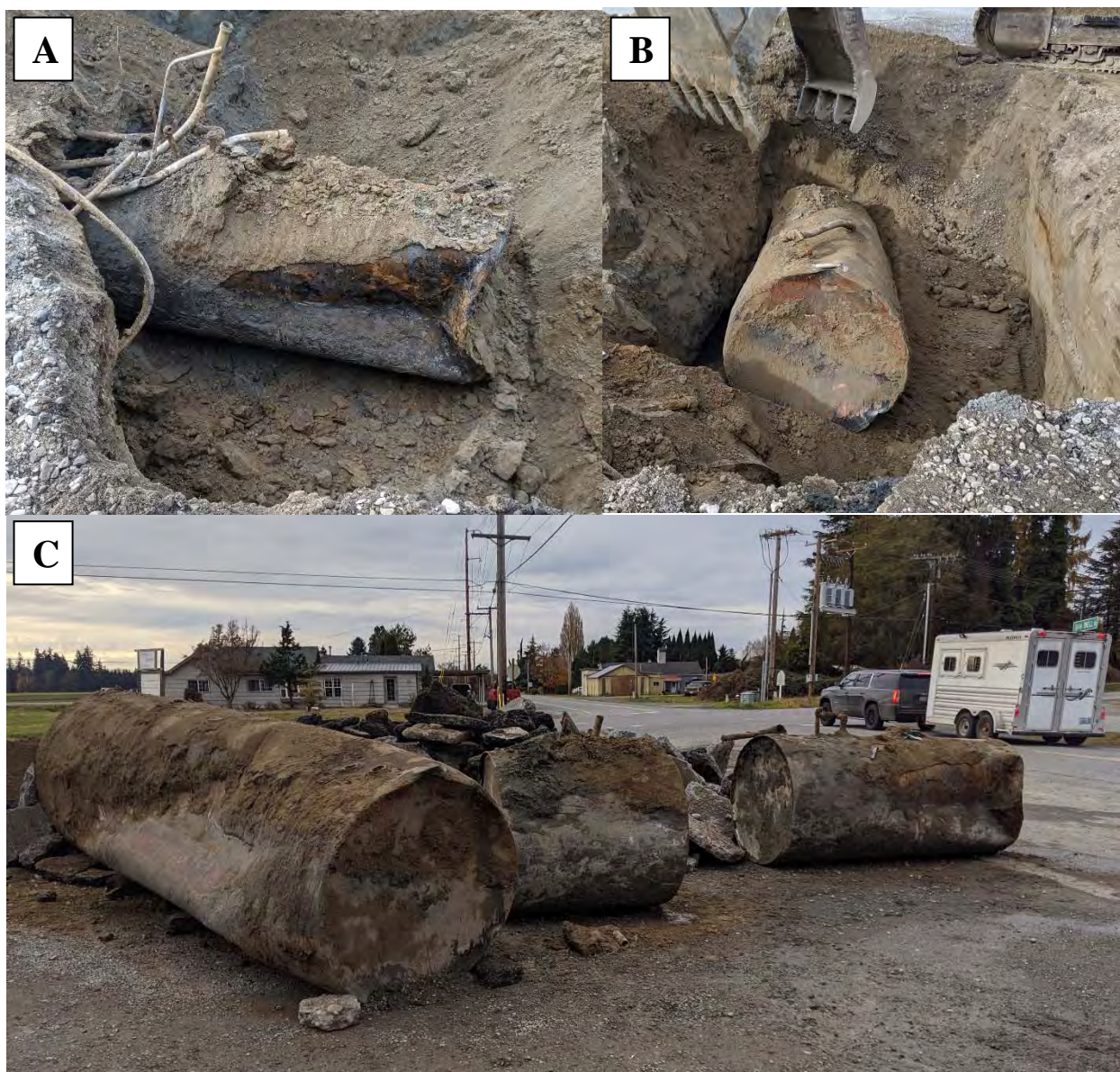
Figure 4. A) Photo of Tank 3 with a significantly rusted exterior. B) Photo of Tank 1 being removed. C) Photo of all three tanks after being removed from the subsurface.
