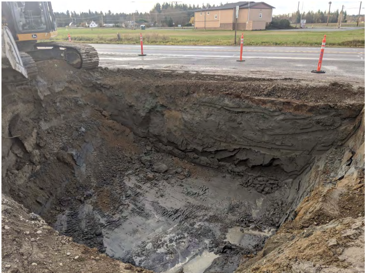
Figure 6. Photo of the UST pit excavation, near completion
