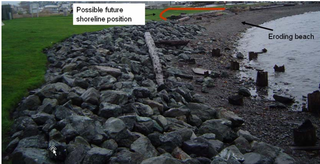
Figure 5. Existing erosional beach and possible future shoreline position (after number of erosion cycles) if no shore protection measures are installed
