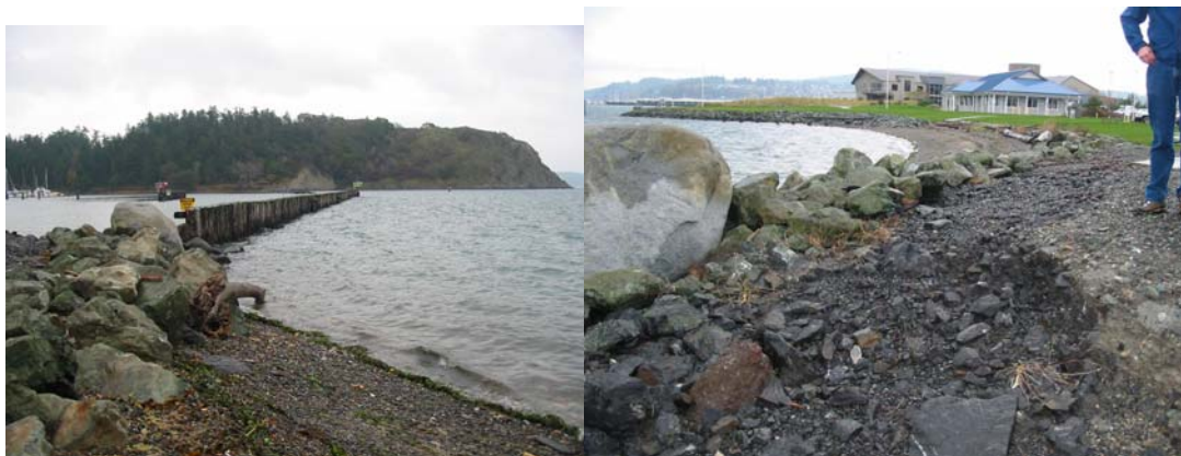
Figure 11. Rock size for shoreline protection at the timber pile wall
