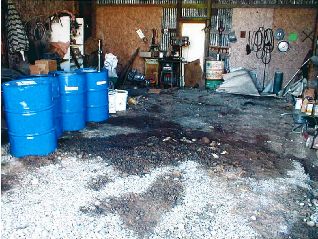
Photo 11: Ground staining within garage.
