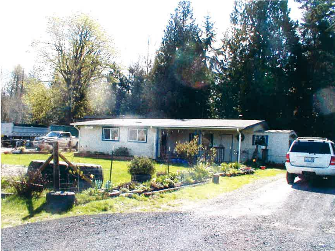
Photo 5: Southeast-facing view of office/residence.
