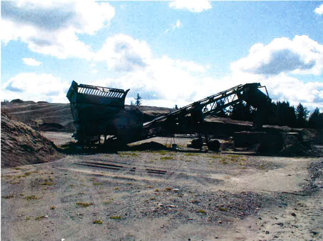
Photo 3: Sifting equipment in center of gravel pit.
