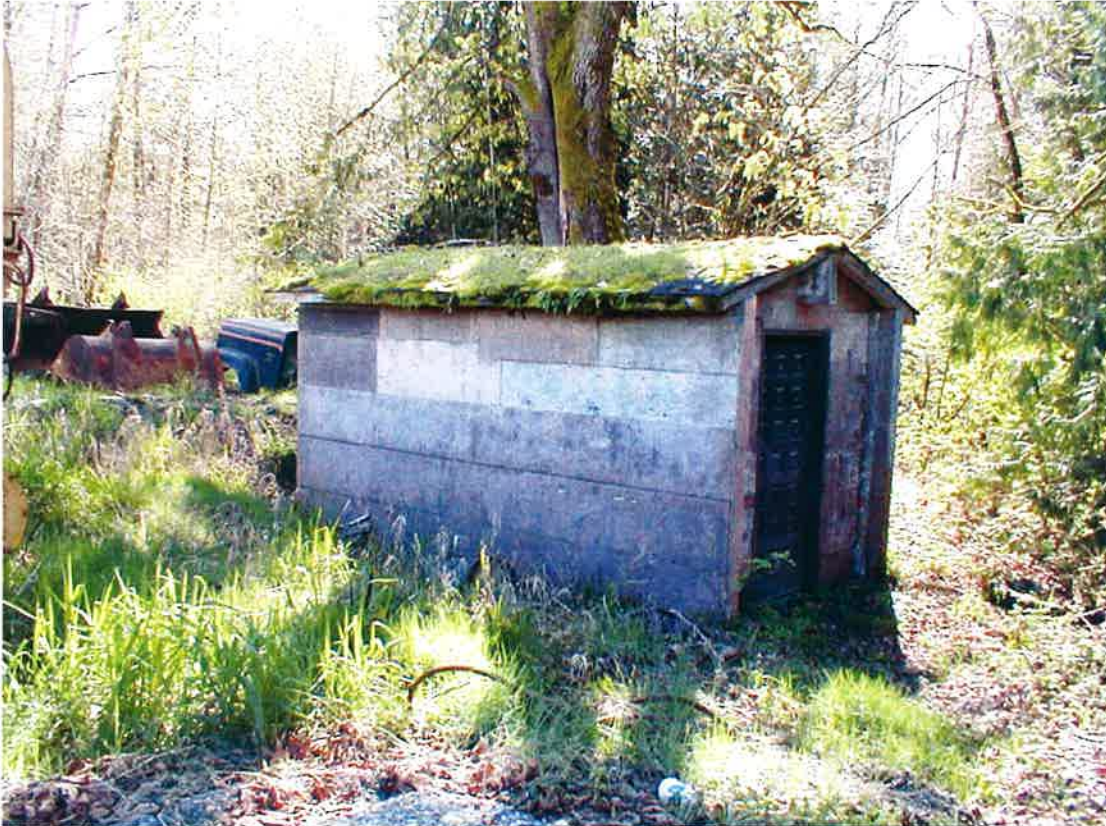
Photo 7: Well house east of office/residence.
