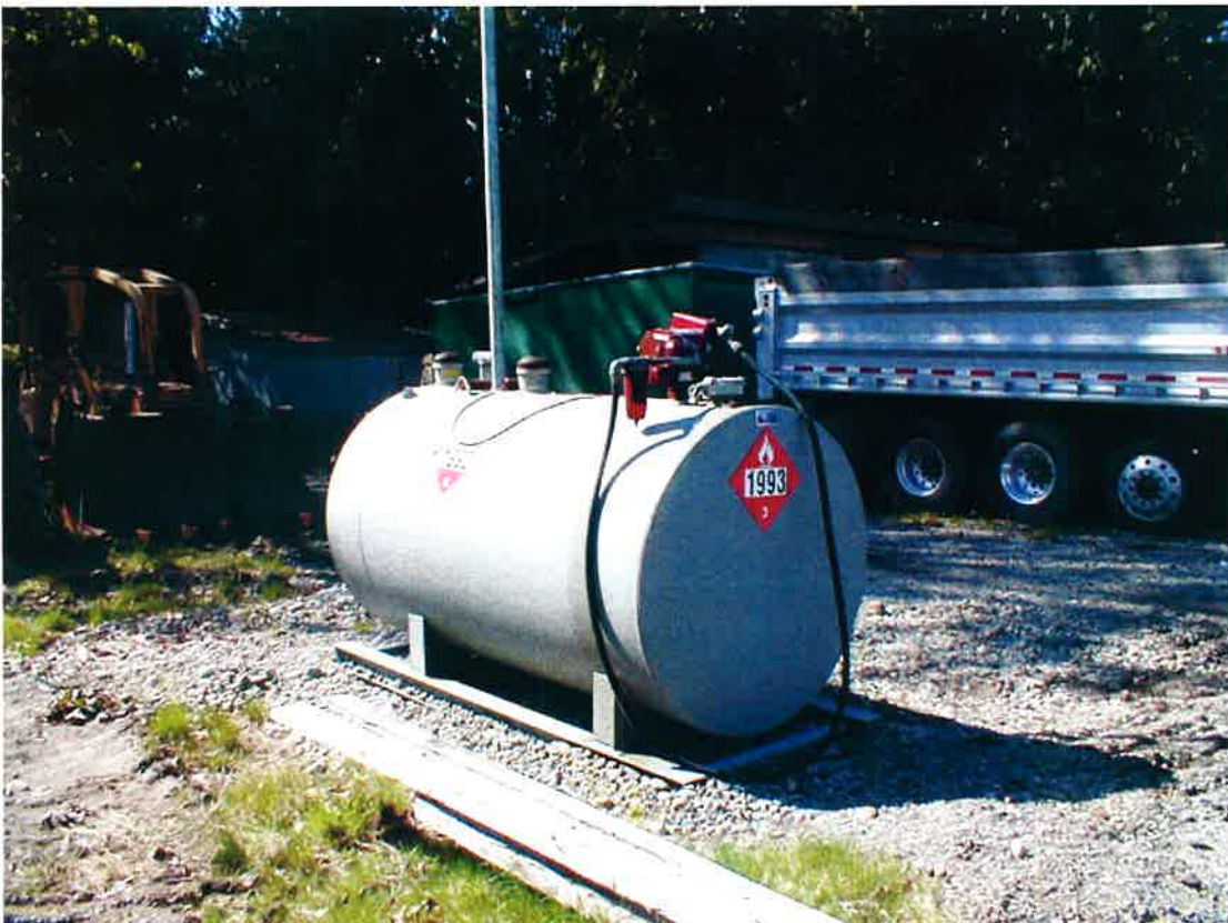
Photo 8: Diesel AST and truck parking near garage.
