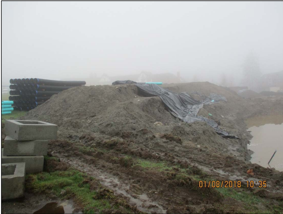
View facing north-northeast showing Stockpile 3 (STK3) – January 8, 2018.
