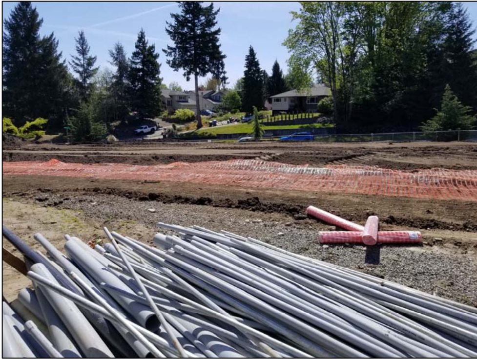
View facing east of modified Type 1 cap- May 1 , 2019.
