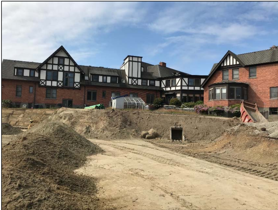
View facing southwest of Bristol View Apartments construction area- June 5, 2018.
