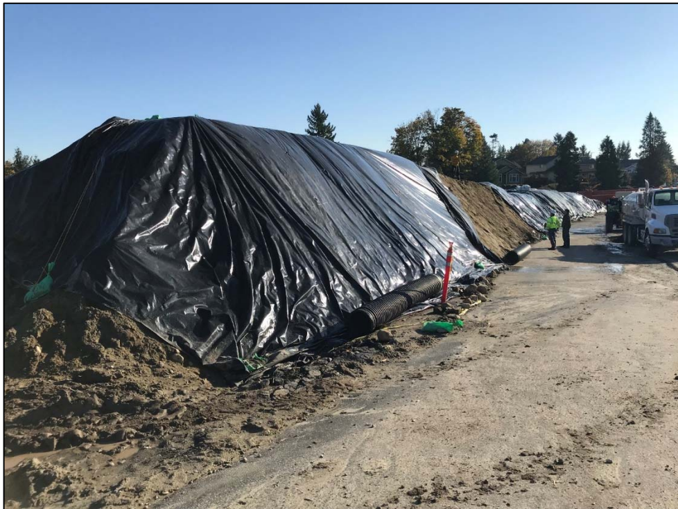
View facing south showing the west-facing slope of Stockpile 1 (STK1) – November 6, 2017.
