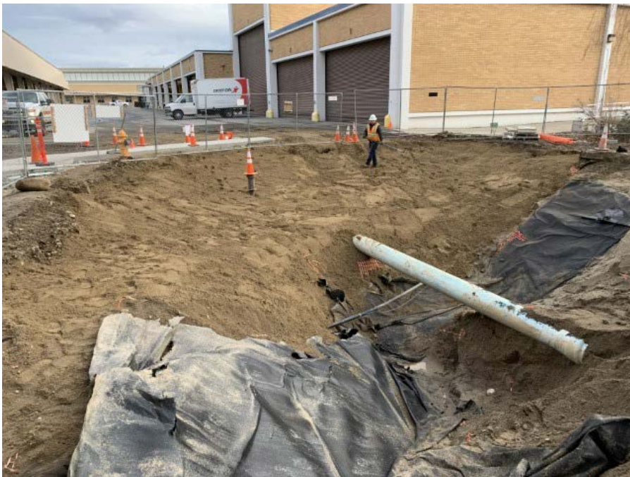
Photograph 8. Bedding sand prepped for geosynthetic liner layout, looking Northeast.
