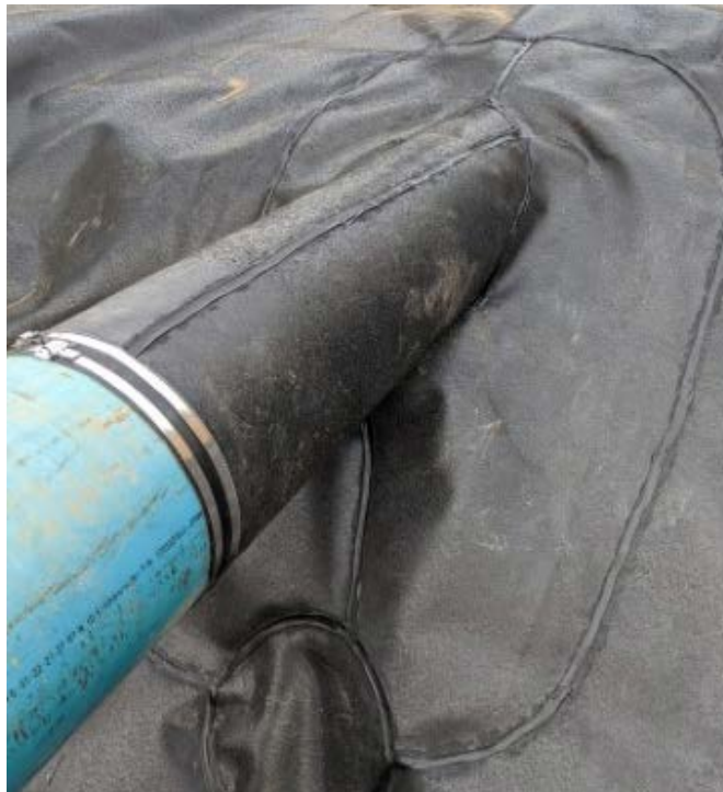
Photograph 11. Welded liner boot around stormwater line, looking North.
