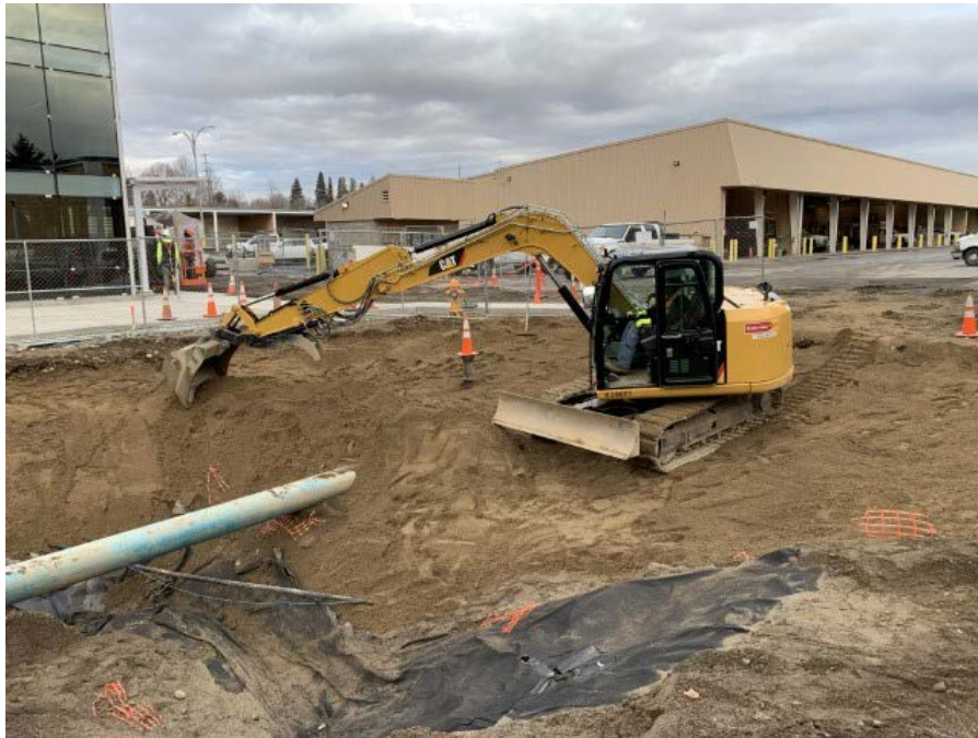
Photograph 7. SES prepares bedding sand for replacement liner section, looking Northwest.
