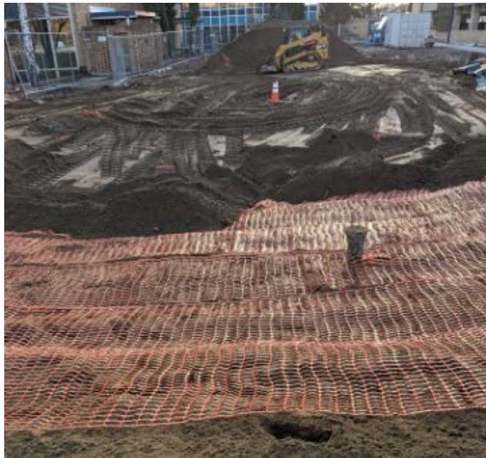
Photograph 20. SES backfills over construction fencing with on-site excavation spoils, looking South.
