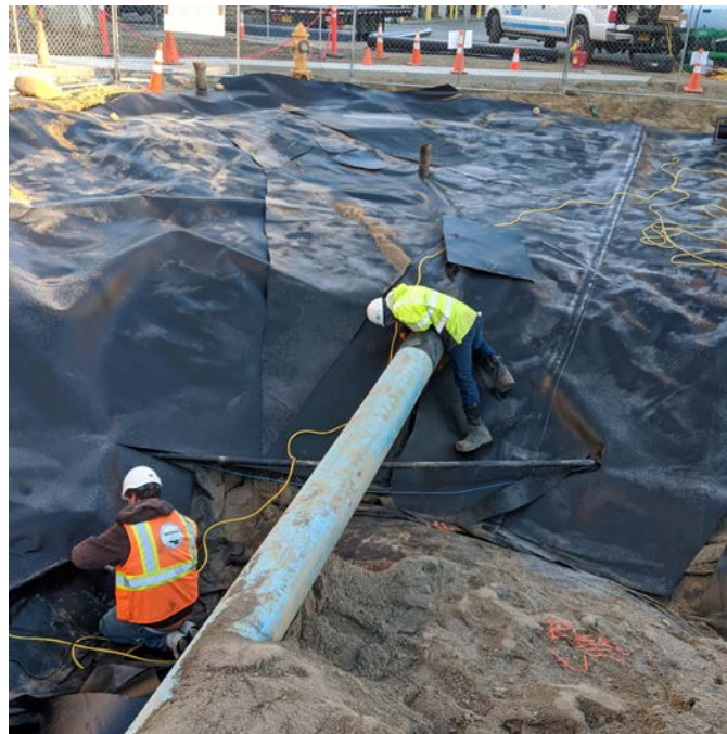
Photograph 10. ACF West welds sections of replacement liner to the existing geosynthetic liner, looking North.
