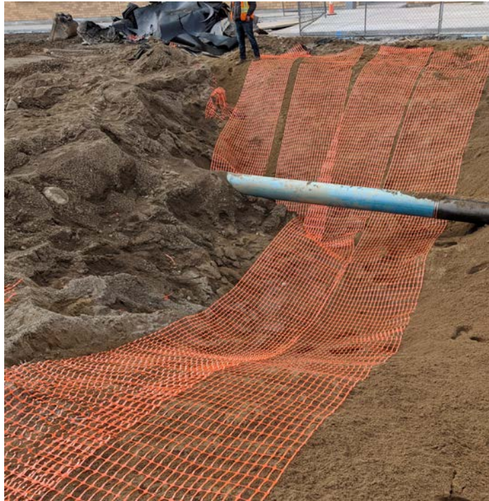
Photograph 19. SES covers bedding sand with orange construction fencing, looking West.
