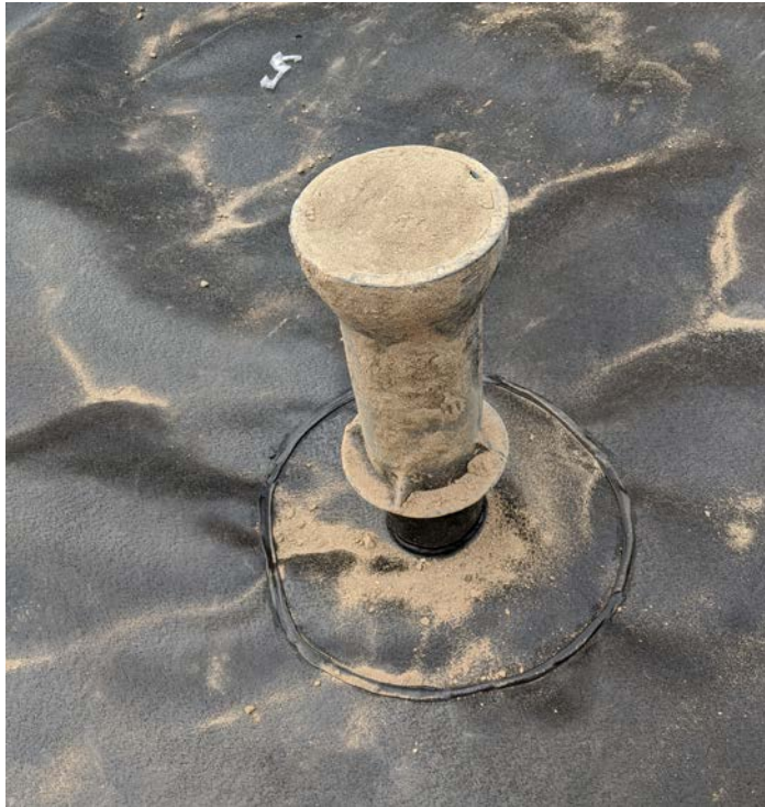
Photograph 14. Welded liner boot around the north water valve stub, looking North.
