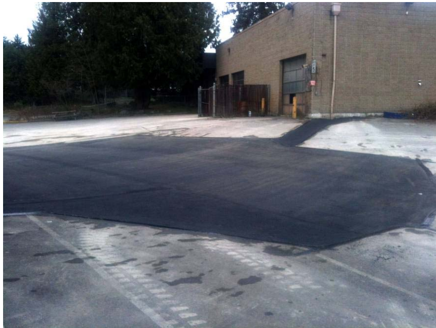
17. Former tank cavity following repaving
