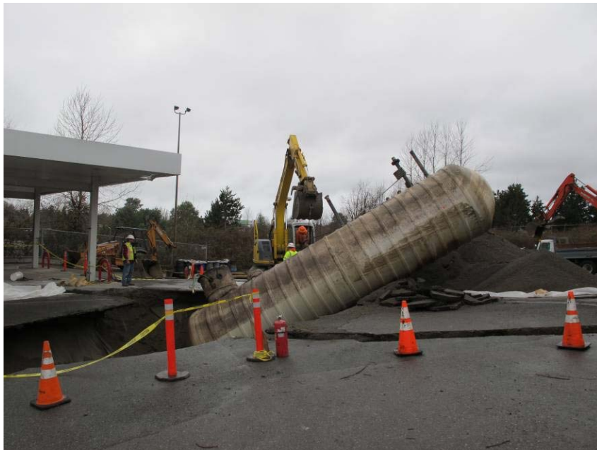
8. 12,000-gallon UST during hoist
