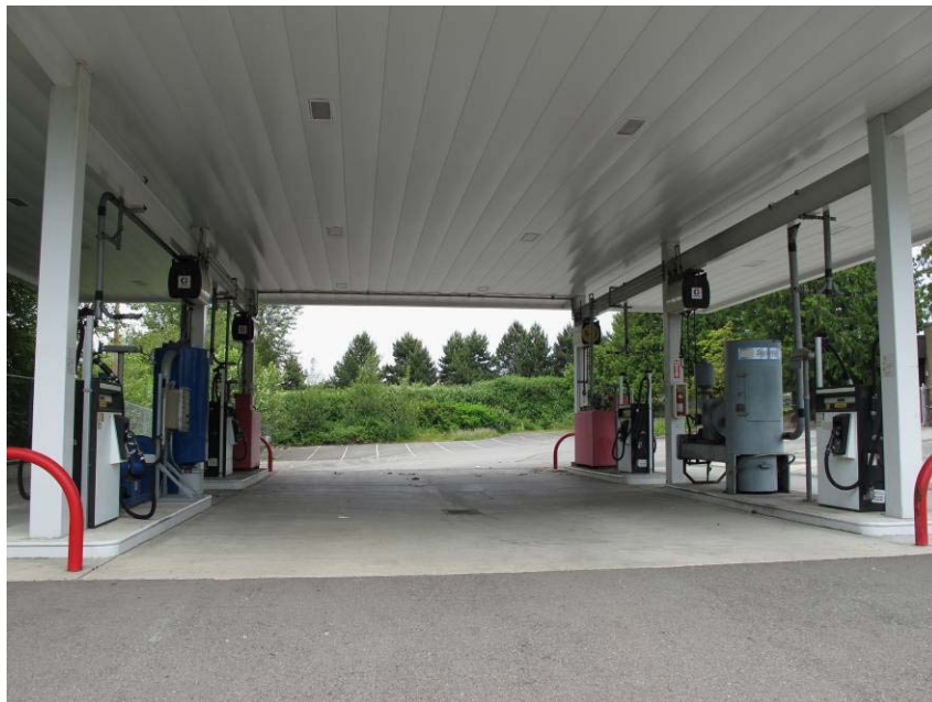
2. Fuel dispenser islands prior to decommissioning
