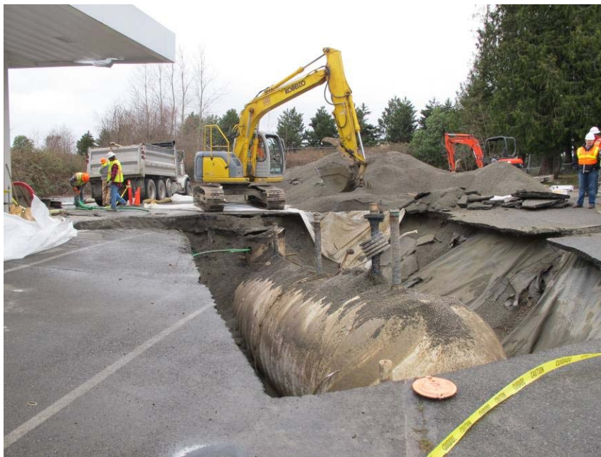
7. 12,000-gallon UST fully uncovered
