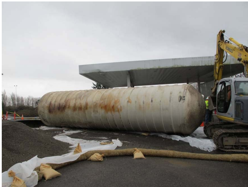
10. Intact 12,000-gallon UST following removal from cavity
