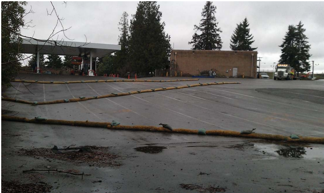
4. Temporary stormwater and erosion controls required by City of SeaTac
