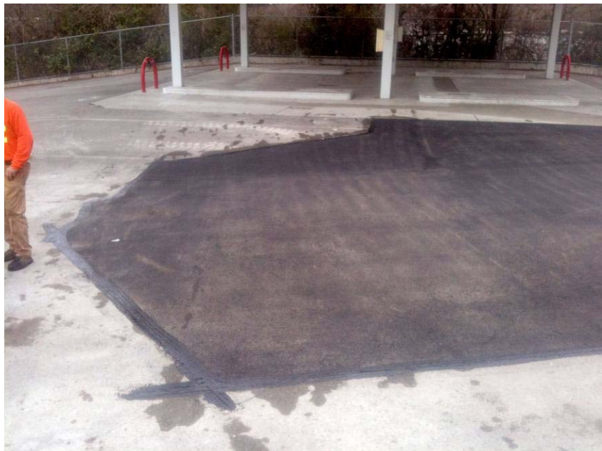
16. Former tank cavity following repaving
