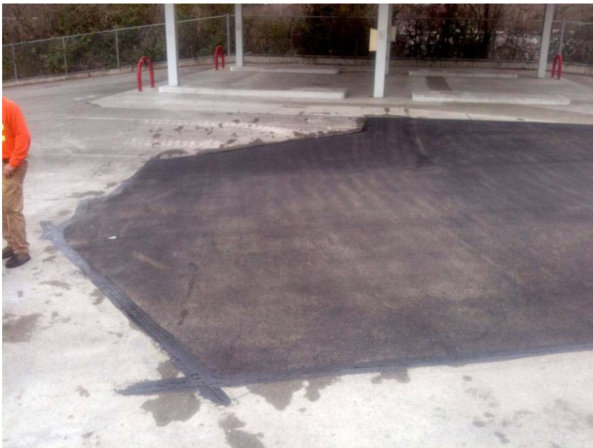
16. Former tank cavity following repaving
