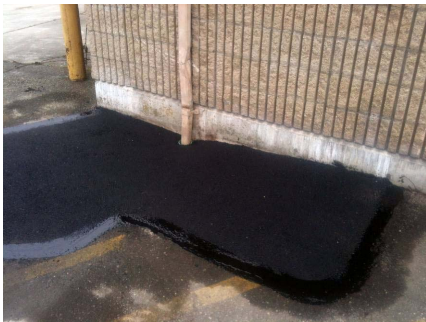
18. Repaved surface near building detail
