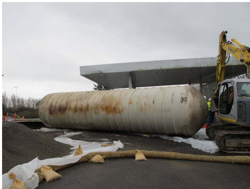
10. Intact 12,000-gallon UST following removal from cavity
