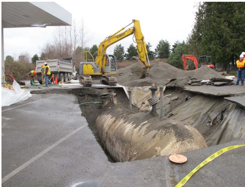
7. 12,000-gallon UST fully uncovered
