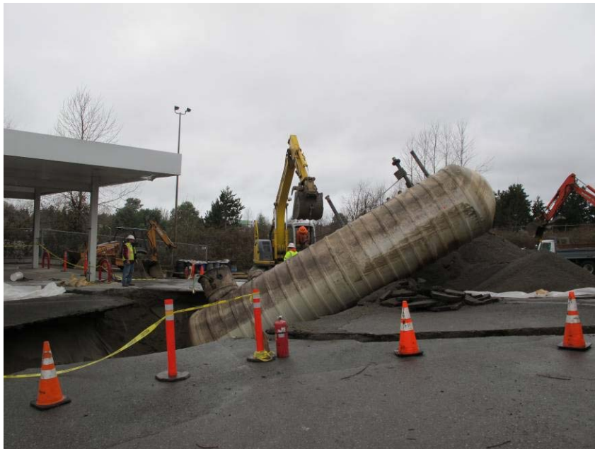
8. 12,000-gallon UST during hoist
