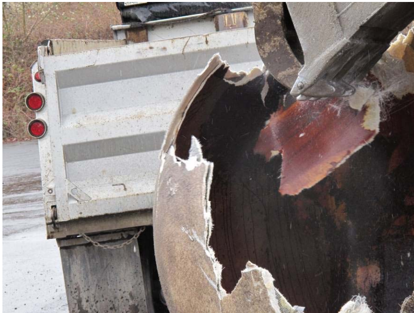
11. On-site crushing of 12,000-gallon fiberglass UST
