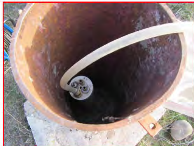
Figure 18: Inside casing view of monitoring well 91AW01 found to contain sample tubing for a submersible pump presumably used by contractors.
