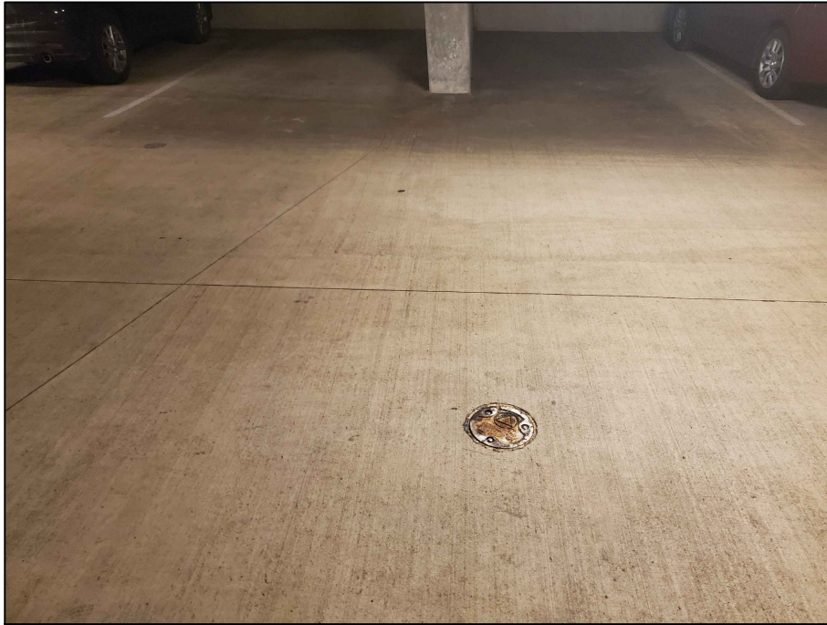
Photograph 7: View looking south at well RW2.
