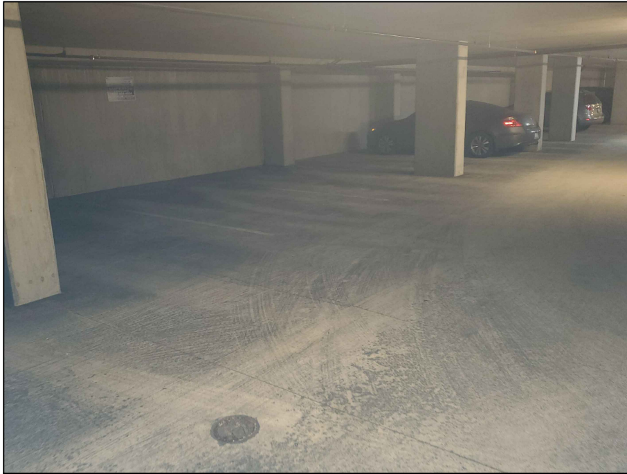
Photograph 1: View looking northwest at the garage floor slab that covers Area 1.
