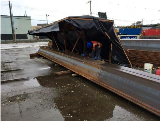
Photograph 7. Shoring wall installation: Adeka sealant application on sheet pile seams. 04/12/18. View facing southwest.
