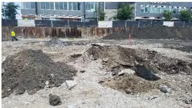
Photograph 11. Pothole sampling locations on the western portion of the property. 06/20/18. View facing north.
