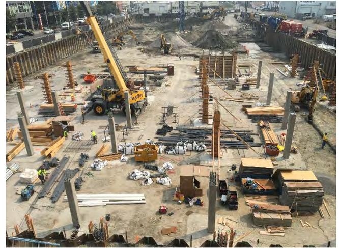
Photograph 18. View of the remedial excavation and new concrete foundation floor poured over final grade on the western portion of the Property in the photo foreground. 08/20/18. View facing east.
