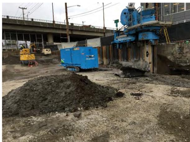
Photograph 14. Removal of north portion of UST01 at the north shoring wall location. 04/11/18. View facing northwest.
