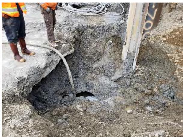
Photograph 13. UST01 location prior to removal, following tank discovery along the north shoring wall. 04/11/18. View facing west.
