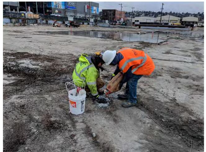
Photograph 4. Licensed driller decommissioning well B-303. 02/23/18. View facing northeast.
