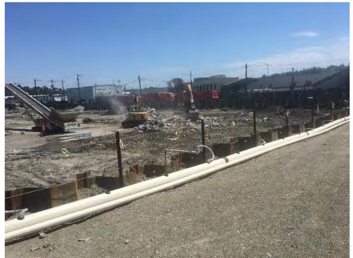
Photograph 10. Concrete slab removal in progress. 06/19/18. View facing southeast.
