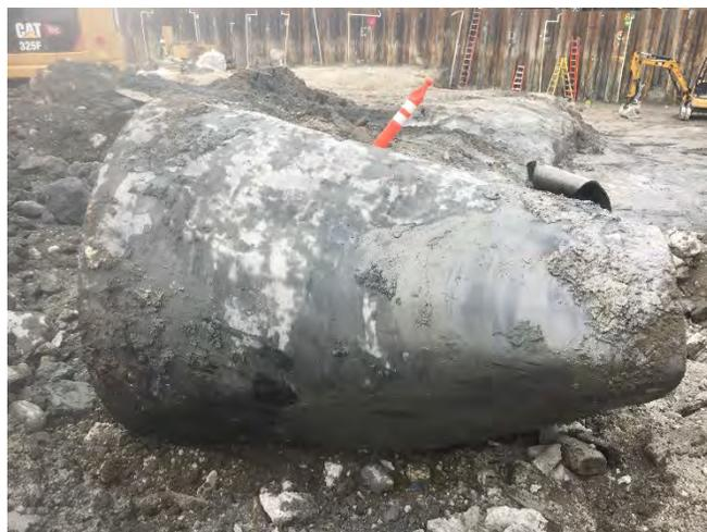
Photograph 16. Scrap metal remnant of decommissioned UST01 following removal. 06/28/18. View facing southwest.
