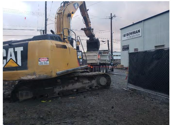
Photograph 20. Loading-out of excavated contaminated soil. 01/07/19. View facing southeast.
