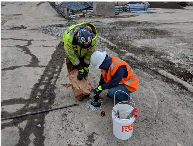
Photograph 3. Licensed driller decommissioning well MW06. 02/23/18. View facing northwest.
