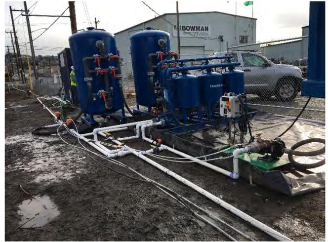
Photograph 2. A portion of the temporary construction stormwater dewatering treatment system. 01/19/18. View facing southeast.
