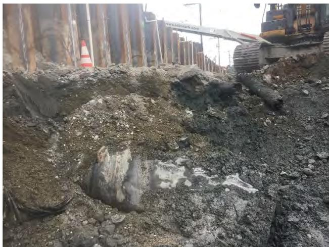
Photograph 15. Removing scrap metal remnant of decommissioned UST01. 06/28/18. View facing east-northeast.
