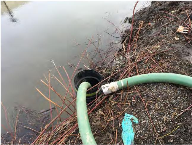
Photograph 1. Temporary dewatering sump, prior to earthwork construction activities. 01/19/18. View facing northeast.
