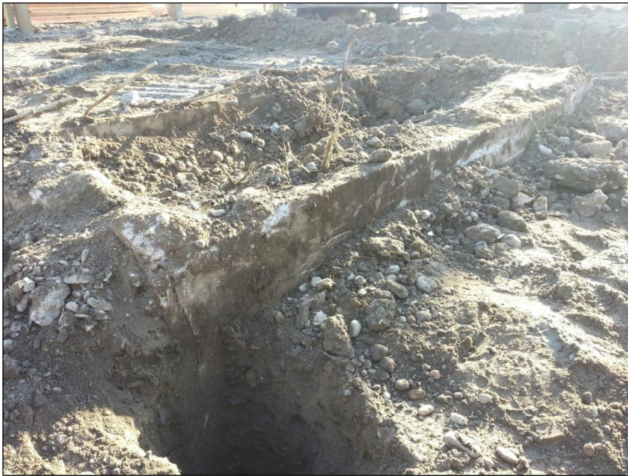
3. Concrete vault structure encountered during the interim action soil removal activities.
