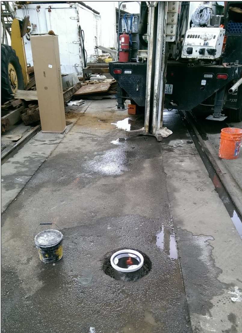
5. WM-MW-4. Typical groundwater monitoring well completion in progress in foreground. Direct-push probe rig used for well installation shown in background.
