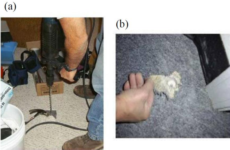
Figure 9. (a)Drilling through a slab, and (b) inner and outer holes (EPA).
