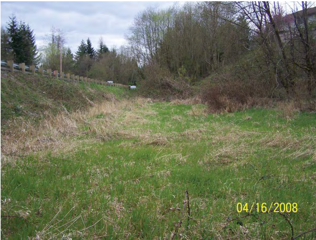
Photo 11. Dry open flat basin west of ditch for stormwater infiltration and treatment—no mudminnow habitat
