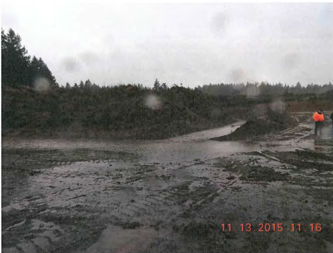
Looking NE—toward soils that were not disturbed by recent site activities.
