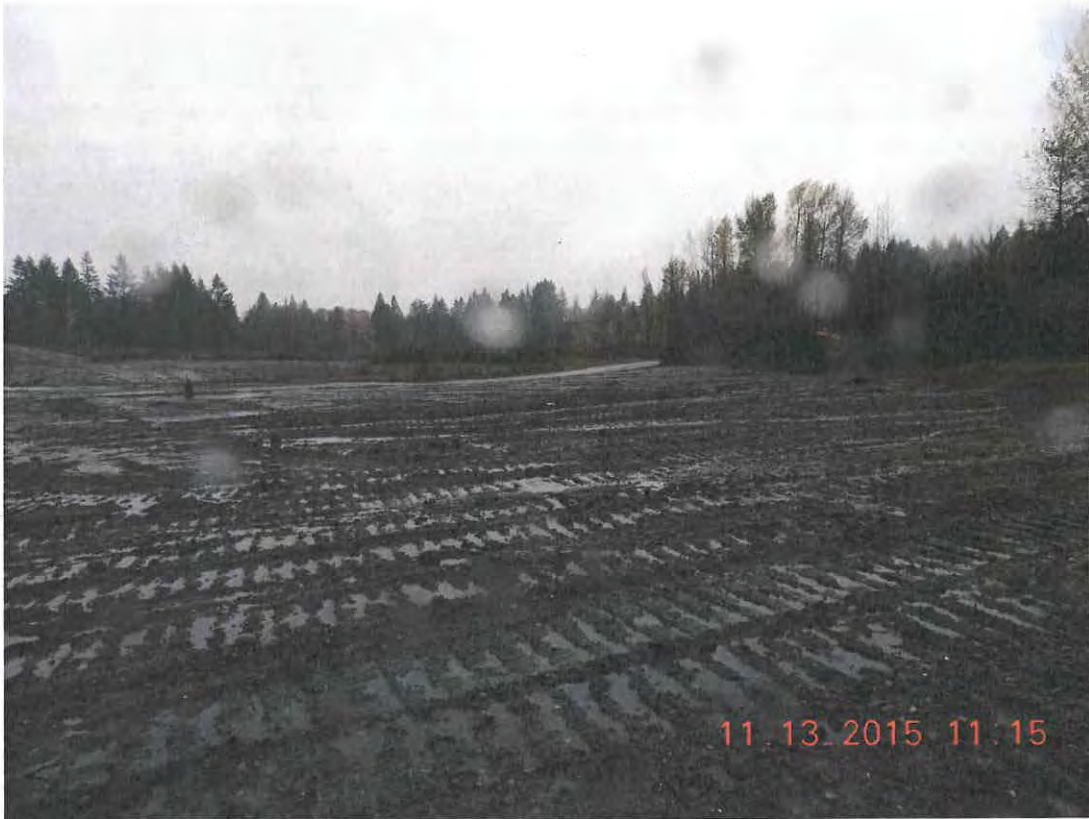
Another view of graded imported soils.
