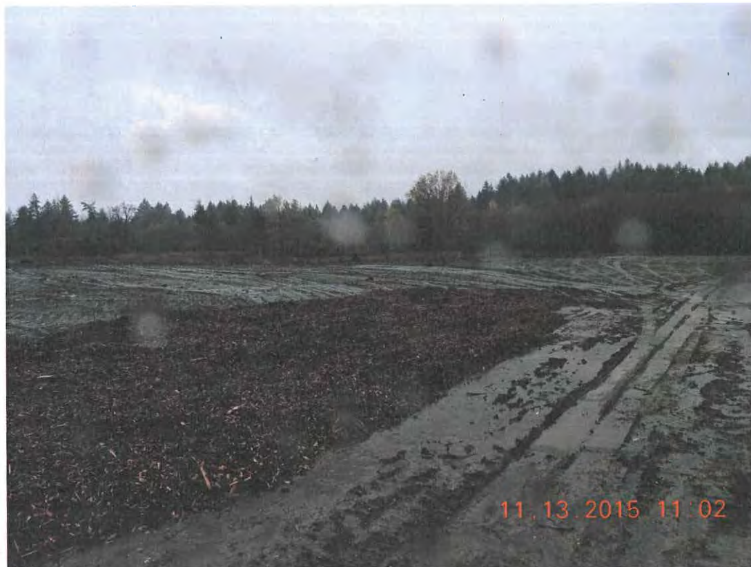
Another view of graded site—wood chips acting as erosion control
