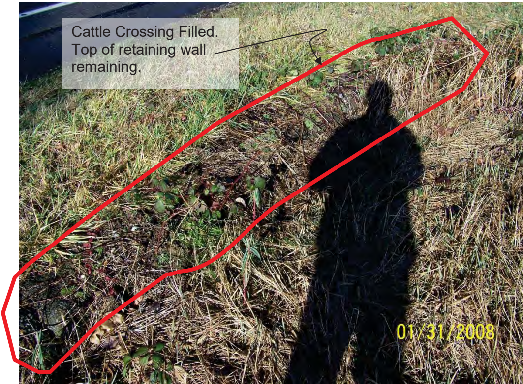
Photo 16. Remnant of filled in cattle tunnel across Cooper Point Road from subject property
