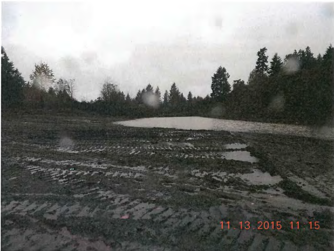
Looking north, toward edge of property—ponded water in old pit floor.
