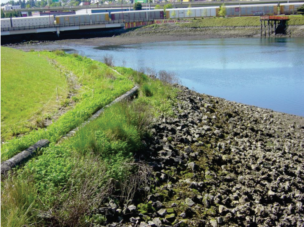
Figure 14 – Looking South at East Bank Slope of the Waterway
