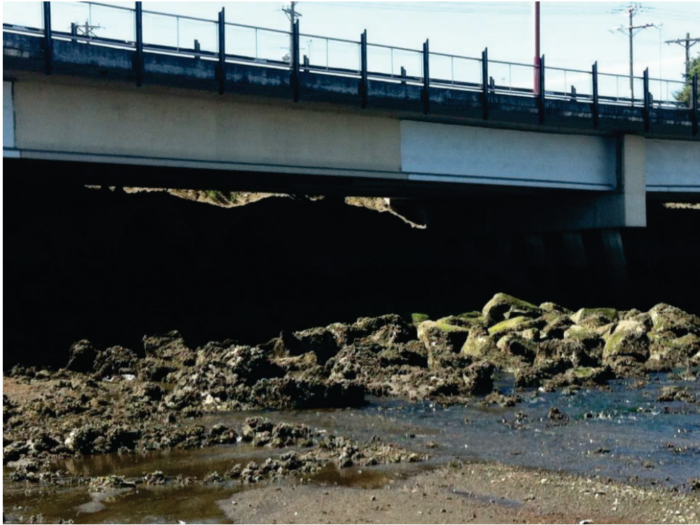
Figure 17 – Looking Southwest at Twin 96-inch Outfalls – Outfalls 237A and 237B
