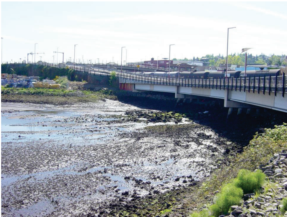
Figure 16 – Looking Southeast at Scour Apron at the Head of the Waterway
