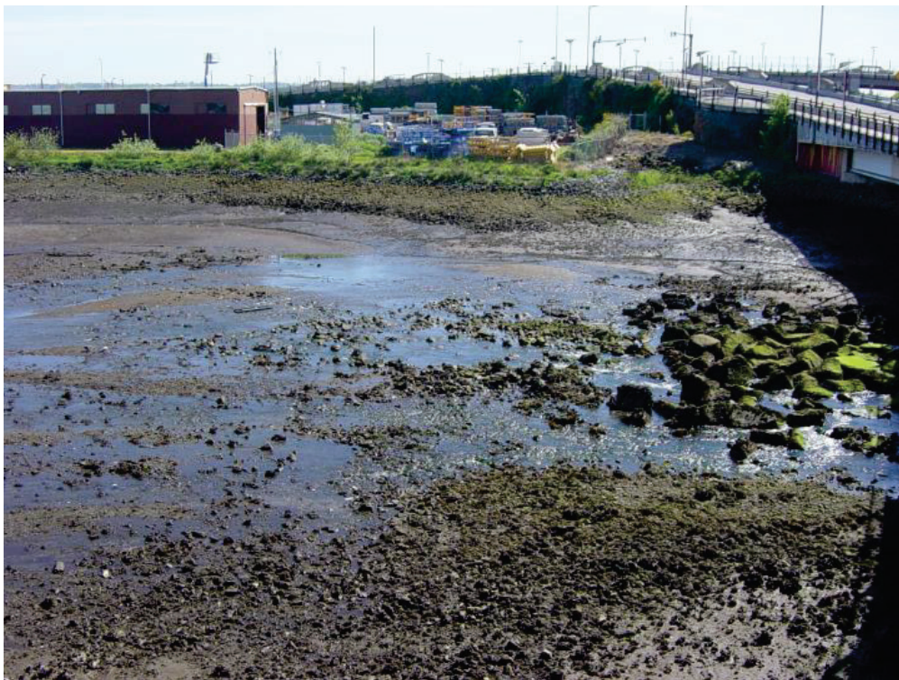
Figure 19 – Looking East across the Scour Apron
