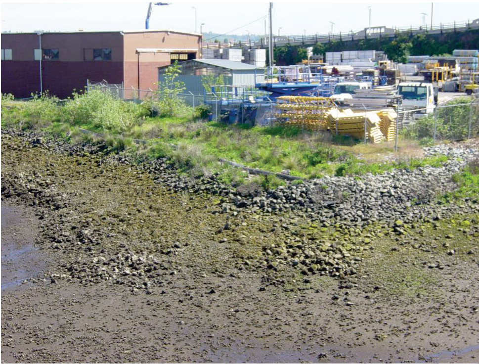
Figure 24 –Former American Plating Site Upland Remediation Completed and in Operation
