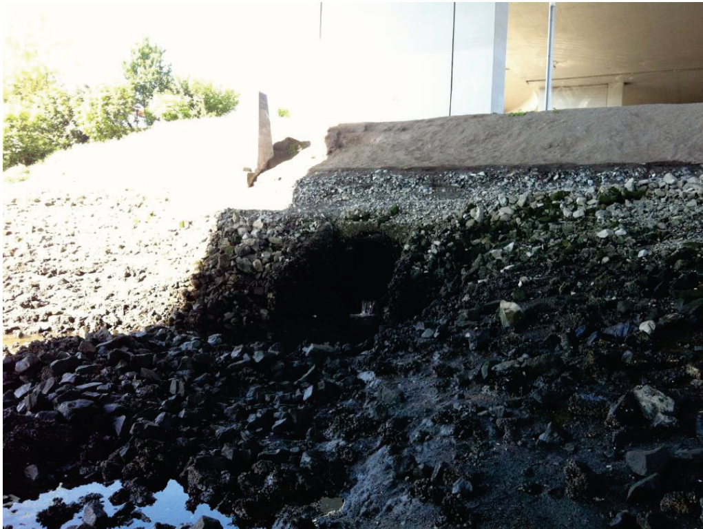
Figure 7 – Outfall #235 Outfall Protection and Flow
