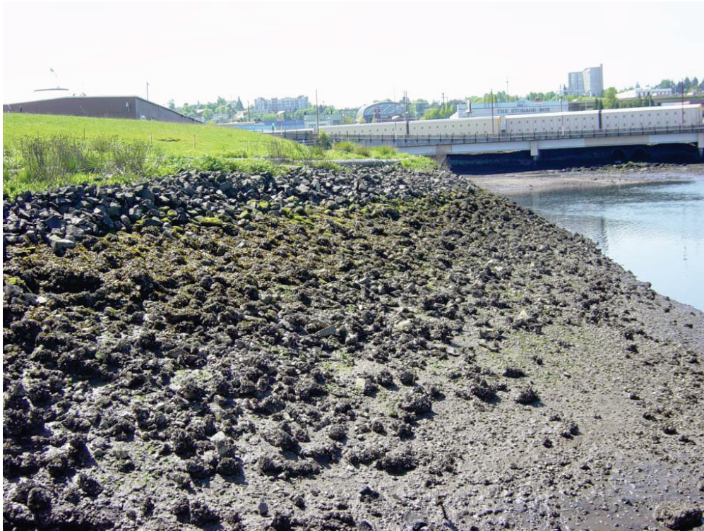
Figure 15 – West Bank Slope of the Waterway
