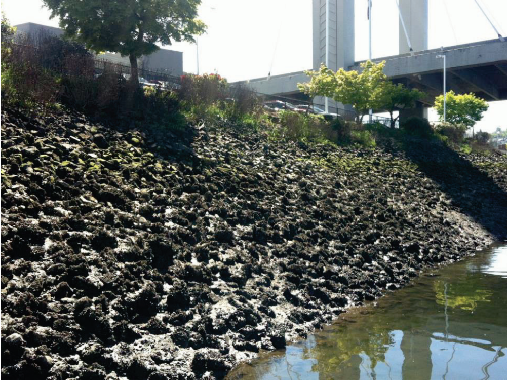
Figure 13 – Looking Southeast at East Bank Slope of the Waterway
