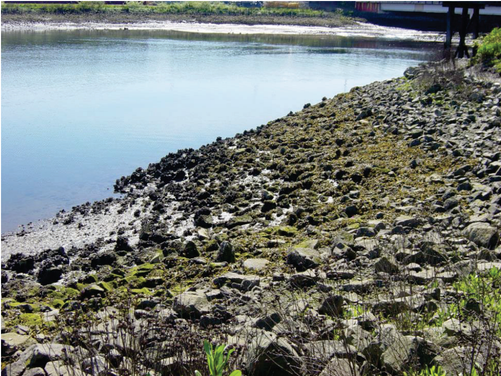
Figure 12 – Looking Southeast at West Bank Slope of the Waterway
