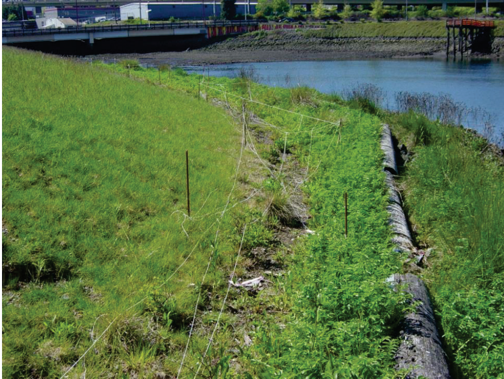
Figure 22 – Former American Plating Site Upland Remediation Area
