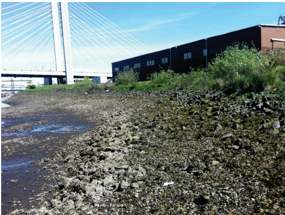
Figure 27 – Looking Northeast at Stormwater Outfalls on East Bank Slope
