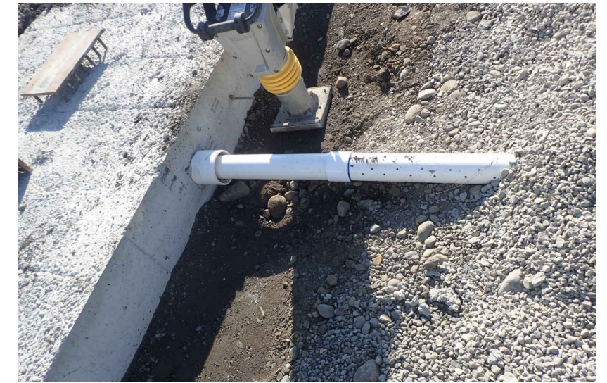
TYPICAL COLLECTION PIPE TROUGH GRADE BEAM PHOTO
