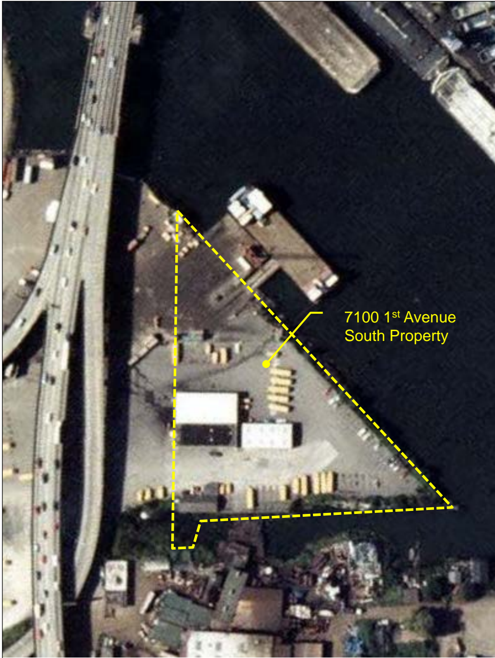
Photograph #4. Circa 1984 aerial photograph showing the 7100 LLC Site and surrounding area along the Lower Duwamish Waterway.
