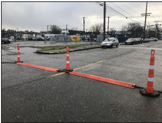
Photo 3: Hose ramps and cones for traffic control around the water hose.
