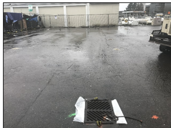
Photo 6: Drains blocked so surfacing and product leaks do not enter the sewers.
