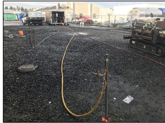
Photo 2: REGENESIS trailer injecting solution into direct push points.
