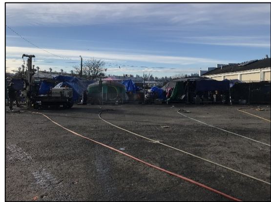
Photo 4: Geoprobe drill rig and injection hoses connected to four direct push points.
