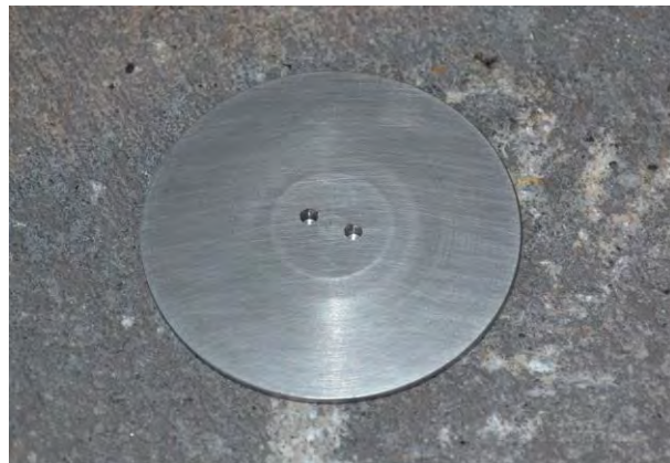
Figure 4. Secure Cover Installed
