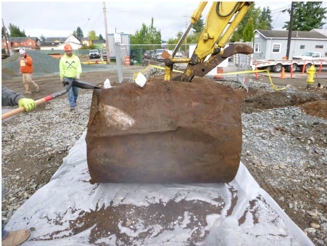
Excavated UST looking west.
