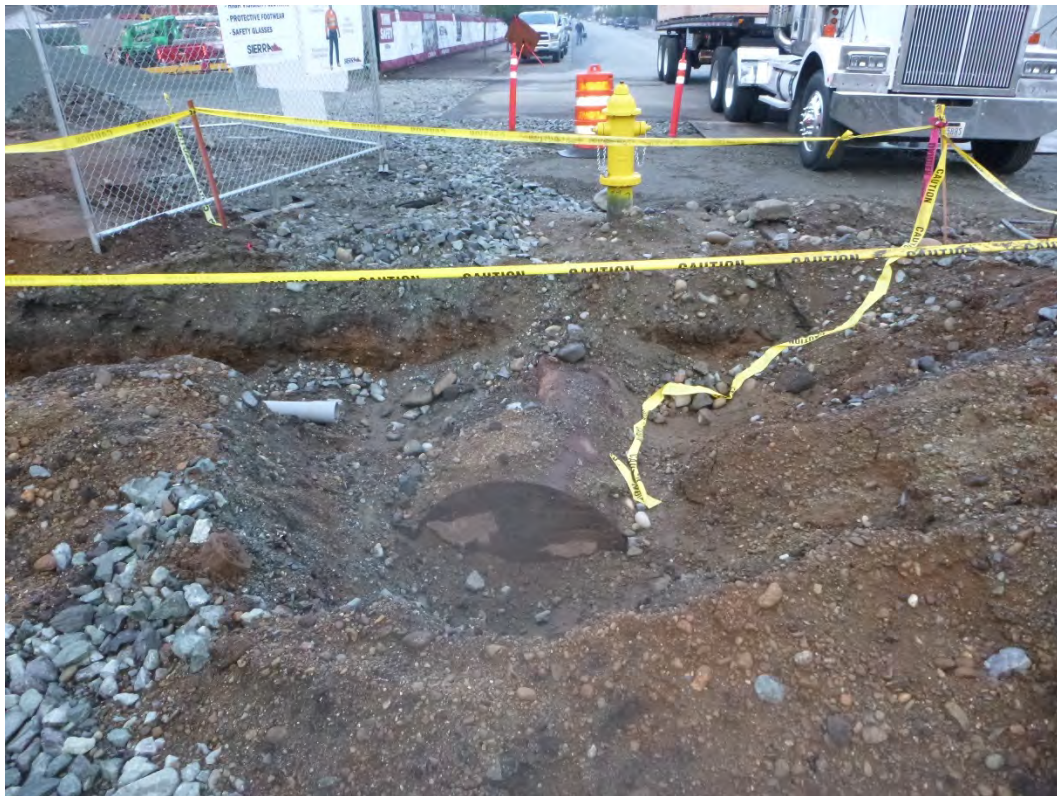
UST in situ looking west.
