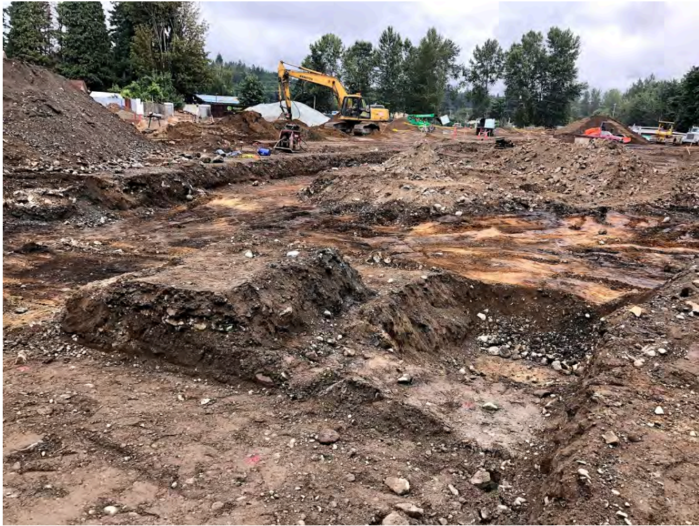
3. Building C and rinse tank area after excavation.
