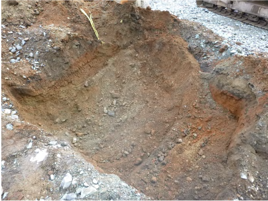
Excavated area looking east.
