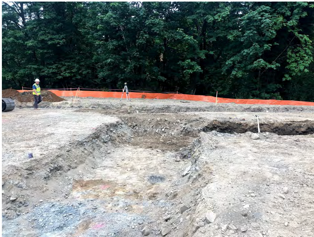
6. Looking south at Building C and rinse tank excavation.
