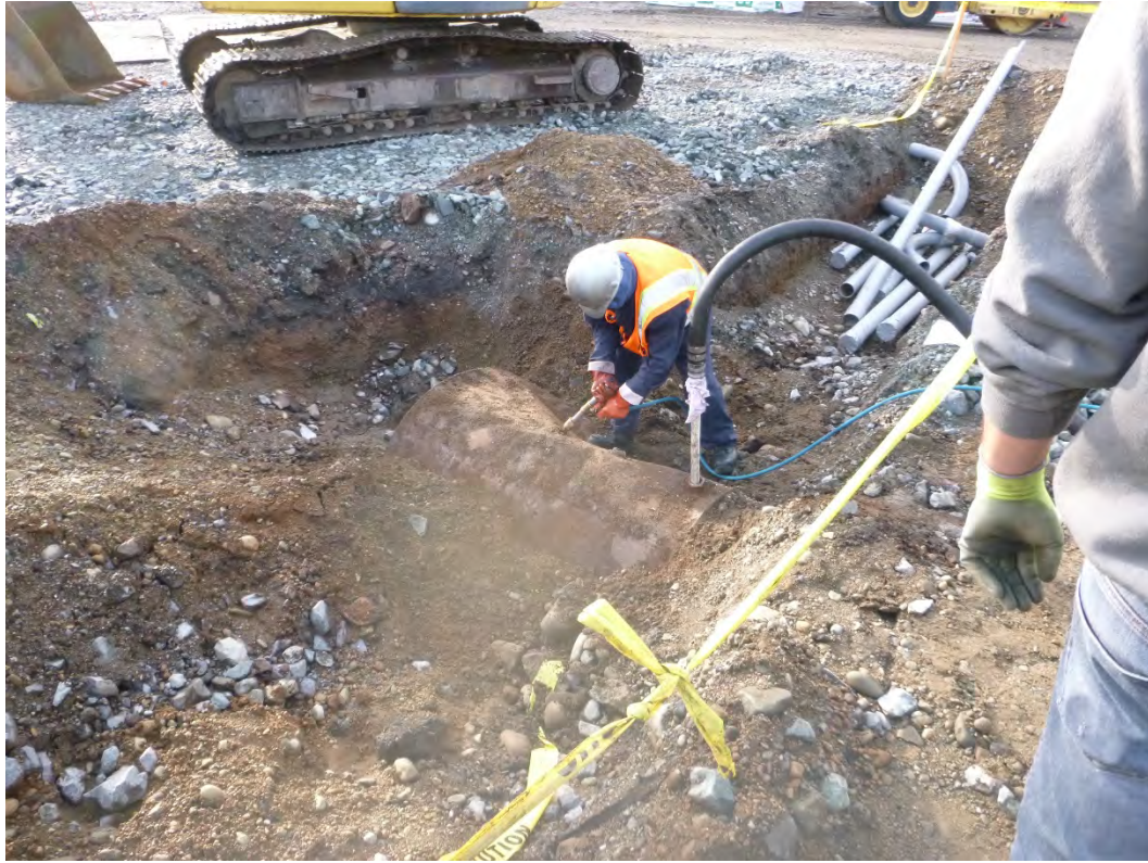
UST decommissioning looking south.
