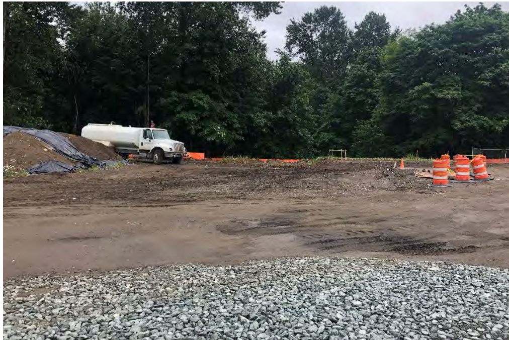
4. Looking south at AOC1 area before excavation.
