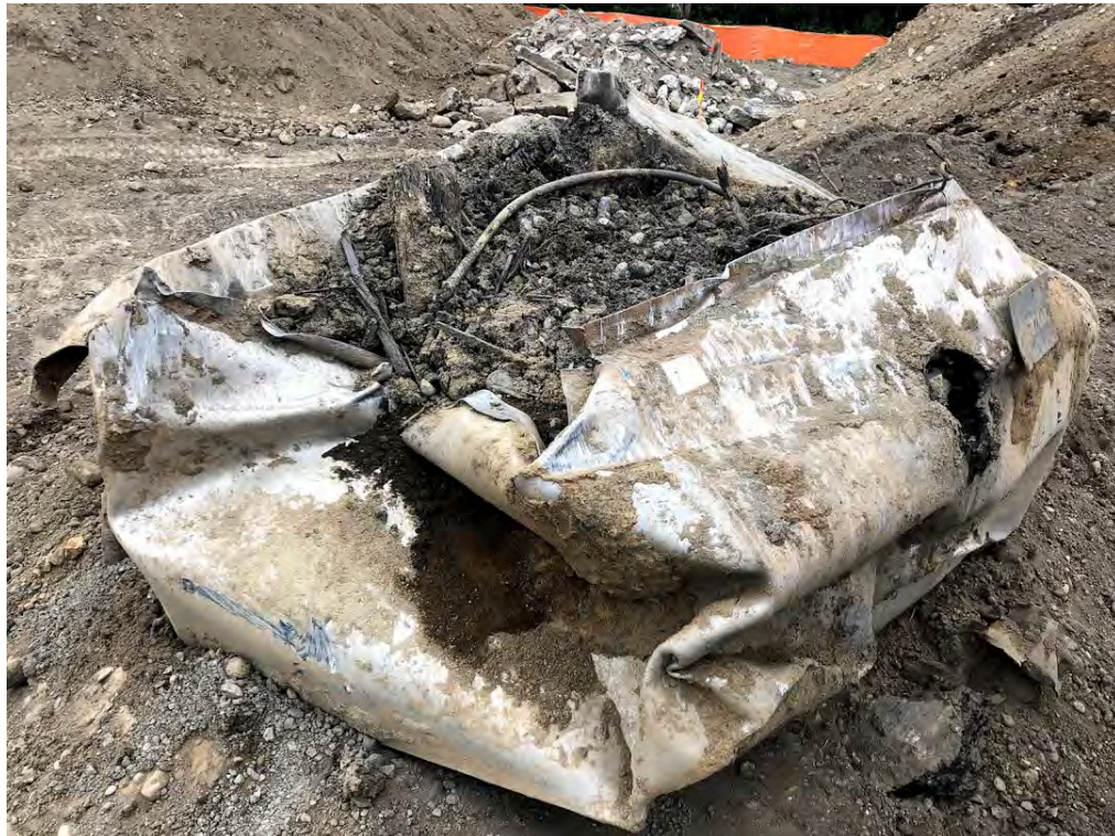
8. Removed rinse tank from Building C area.
