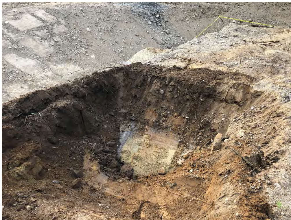
2. AOC3 initial excavation and sidewall sampling location.
