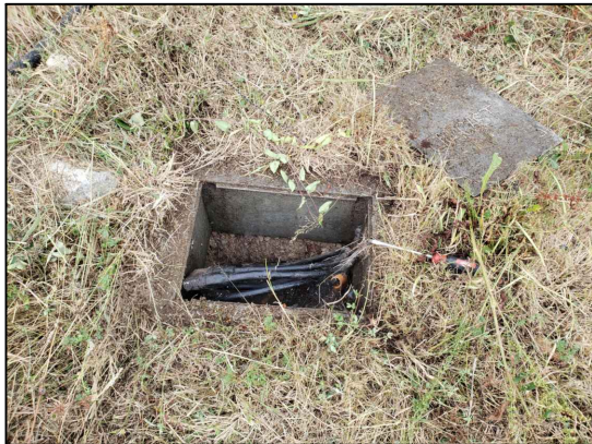
Looking Inside Vault
