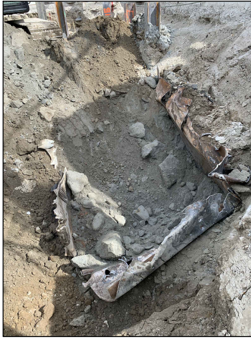
Photograph 7: View of CDF being excavated from inside UST6B.
