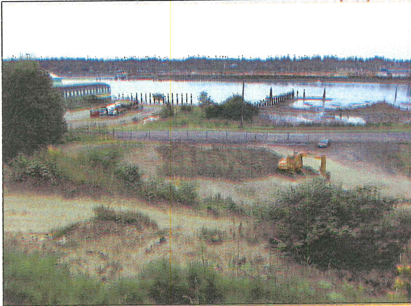
Subject property looking east during excavation
