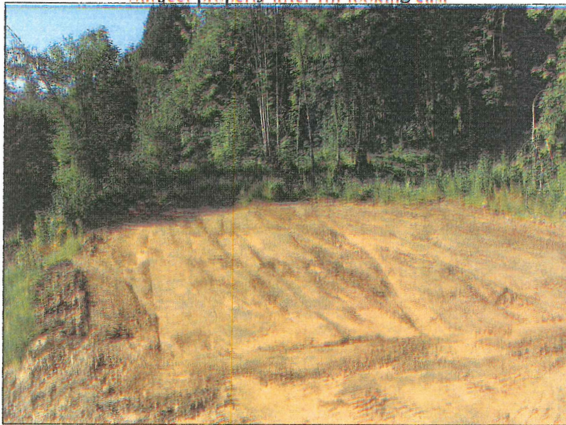
Top of subject property after fill
