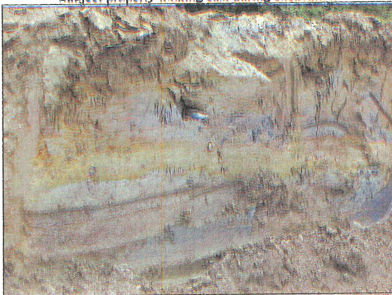
Excavation wall close-up
