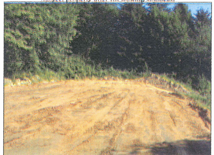
Top of subject property after fill
