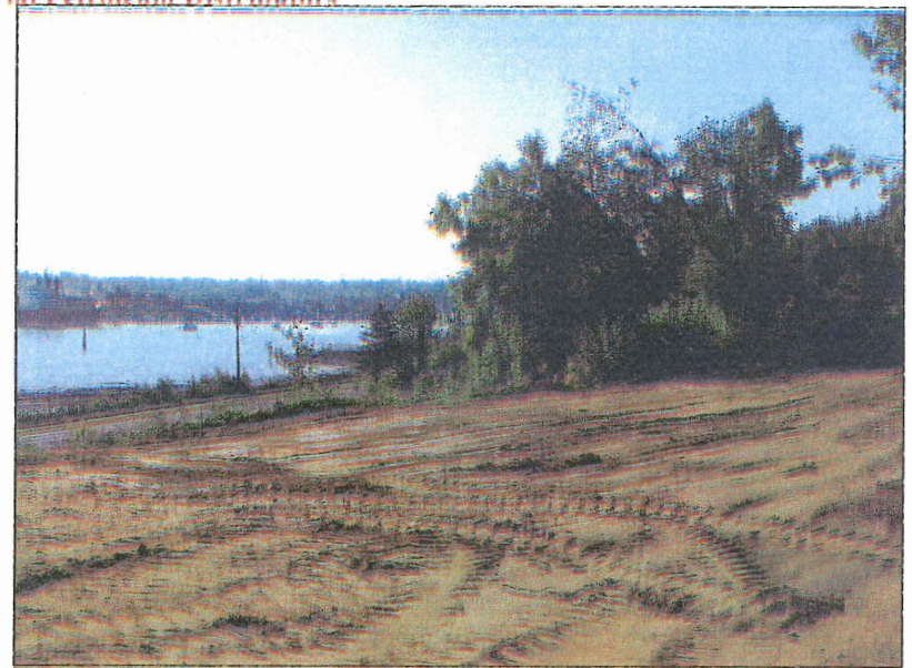
Subject property after fill looking southeast
