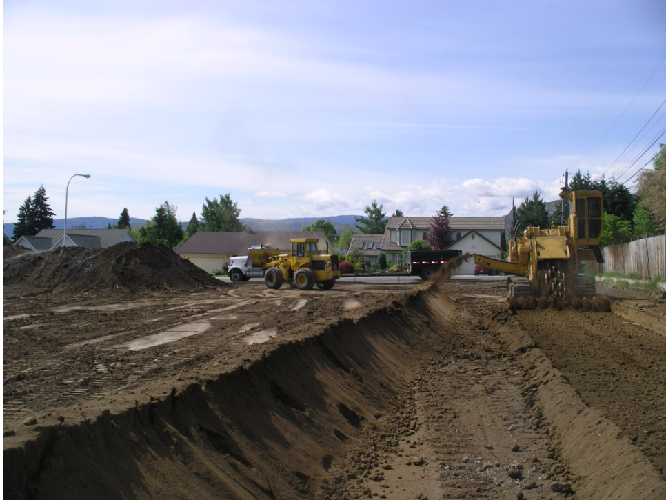
Figure D-1: Deep mixer in action at Lewis & Clark
