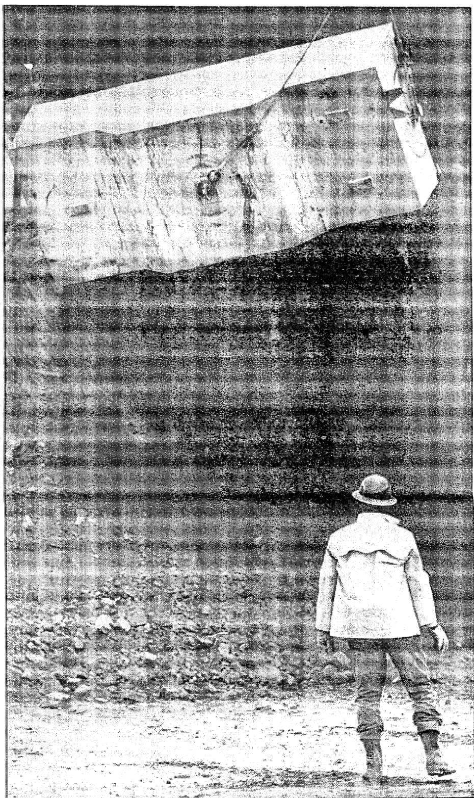
Construction worker John McDonald watches as a load of dirt is dumped. The dirt is removed from Mount Baker Ridge by rail car. The rail cars are lifted by crane and dumped, then the dirt is trucked away.
